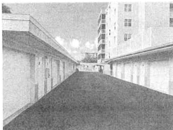
GENERAL VIEW OF GARAGES
