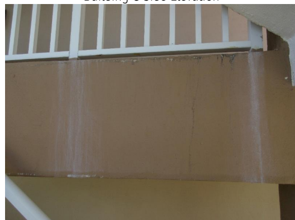
Typical Efflorescence
