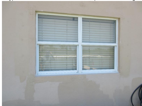
Cracked and Damaged Window Sill Building C
