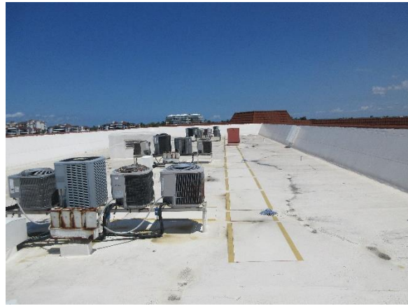
Typical Roof Overview (Bldg A, B, D & E)
