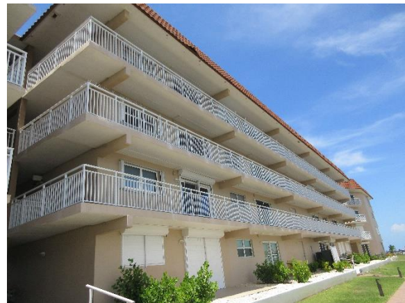
Typical Balcony Railings
