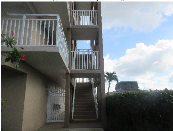
Typical Stair Tower Railings
