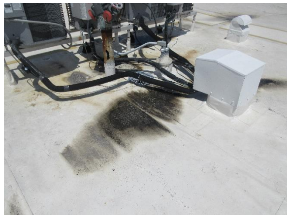
Typical Mechanical Equipment dog-house
