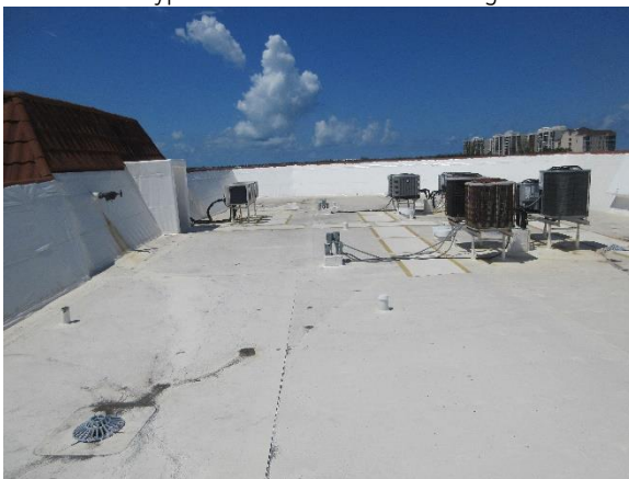
Building C Roof Overview
