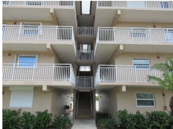
Typical Shared Stair and Walkway (Bldg A, B, D & E)
