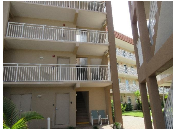
Overview Sample of Residential Windows Replaced
