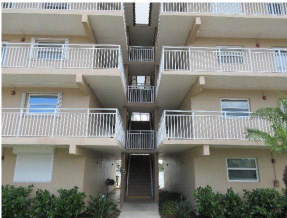
Typical Walkway Railings
