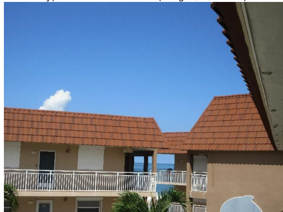
Overview Metal Tile Mansard Roof
