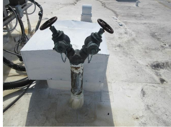
Roof Standpipe
