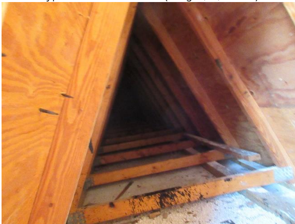
Typical Mansard Roof Framing
