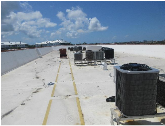
Typical Roof Overview (Bldg A, B, D & E)
