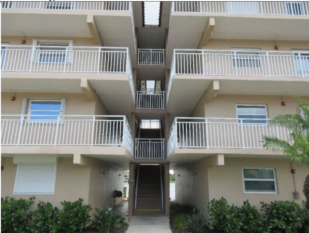
Photo 4. Overview Shared Stair Two and Combined Walkways at Buildings A and B
