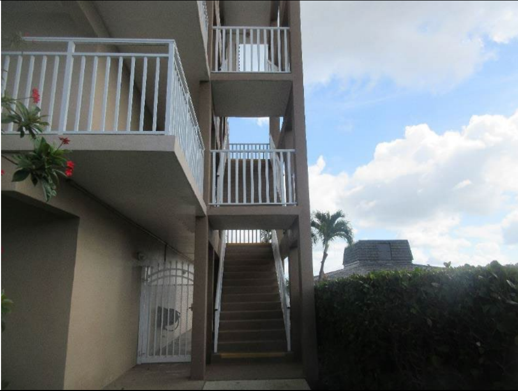
Photo 3. Typical Overview East Side Stair Tower
