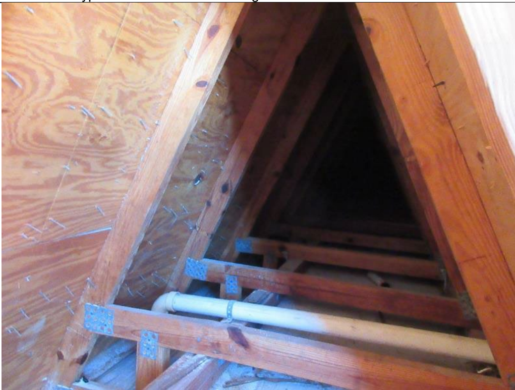
Photo 74. Typical Mansard Roof Framing Building D
