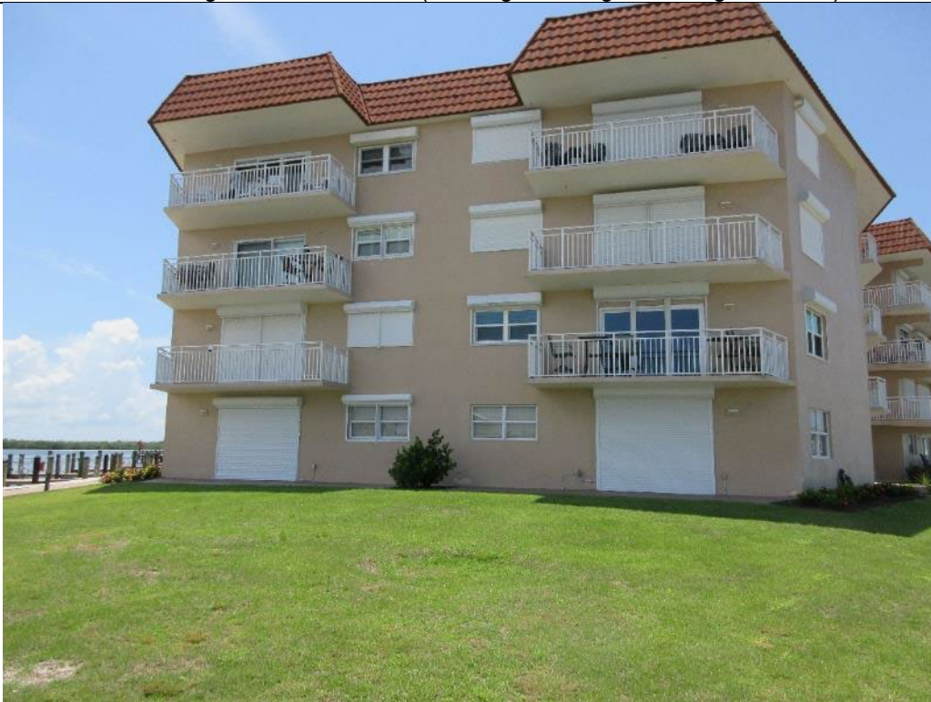
Photo 36. Overview Rear Building C
