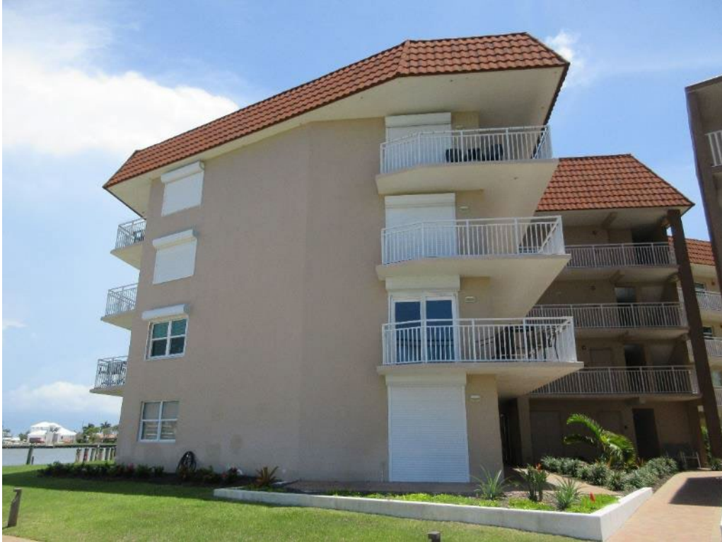
Photo 37. Overview W Elevation Building C Typical Side Balcony and Walkway
