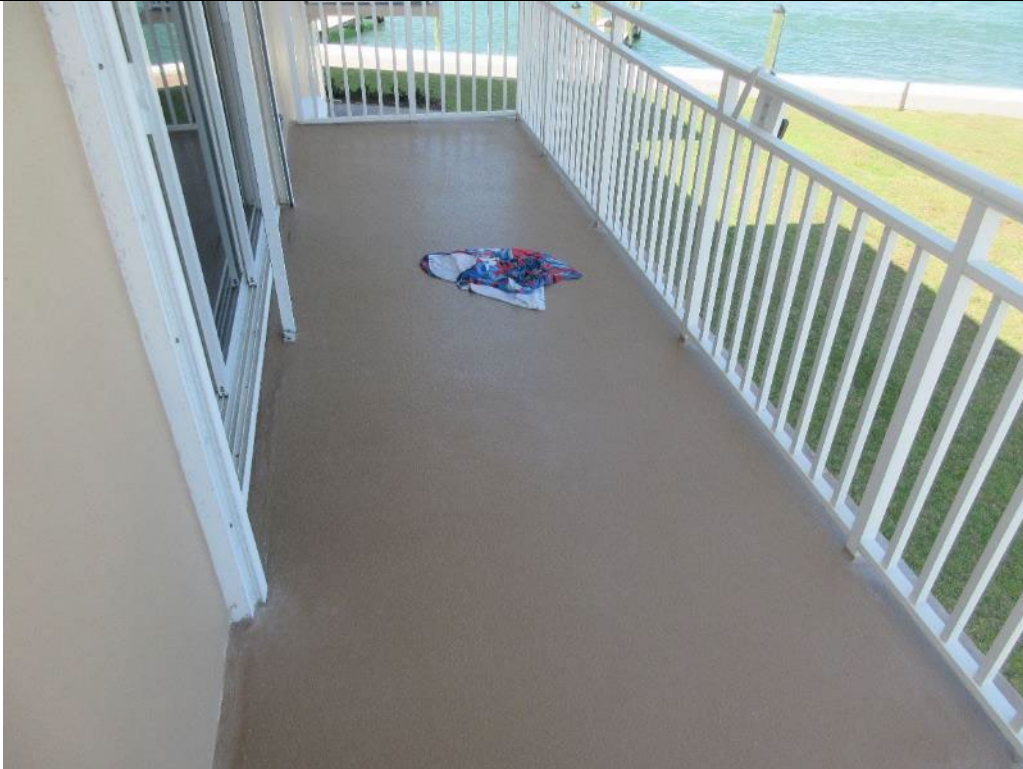
Photo 39. Unit C201 Rear Balcony Overview
