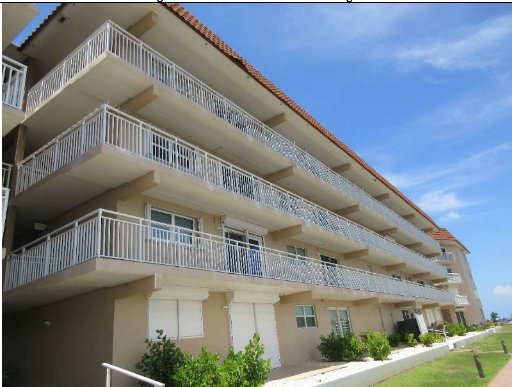
Photo 24. Rear Elevation Building B Overview
