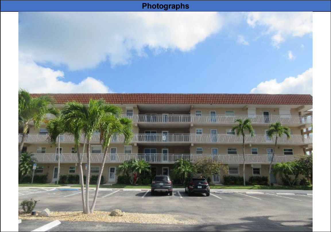
Photo 1. Front Elevation of Building A
