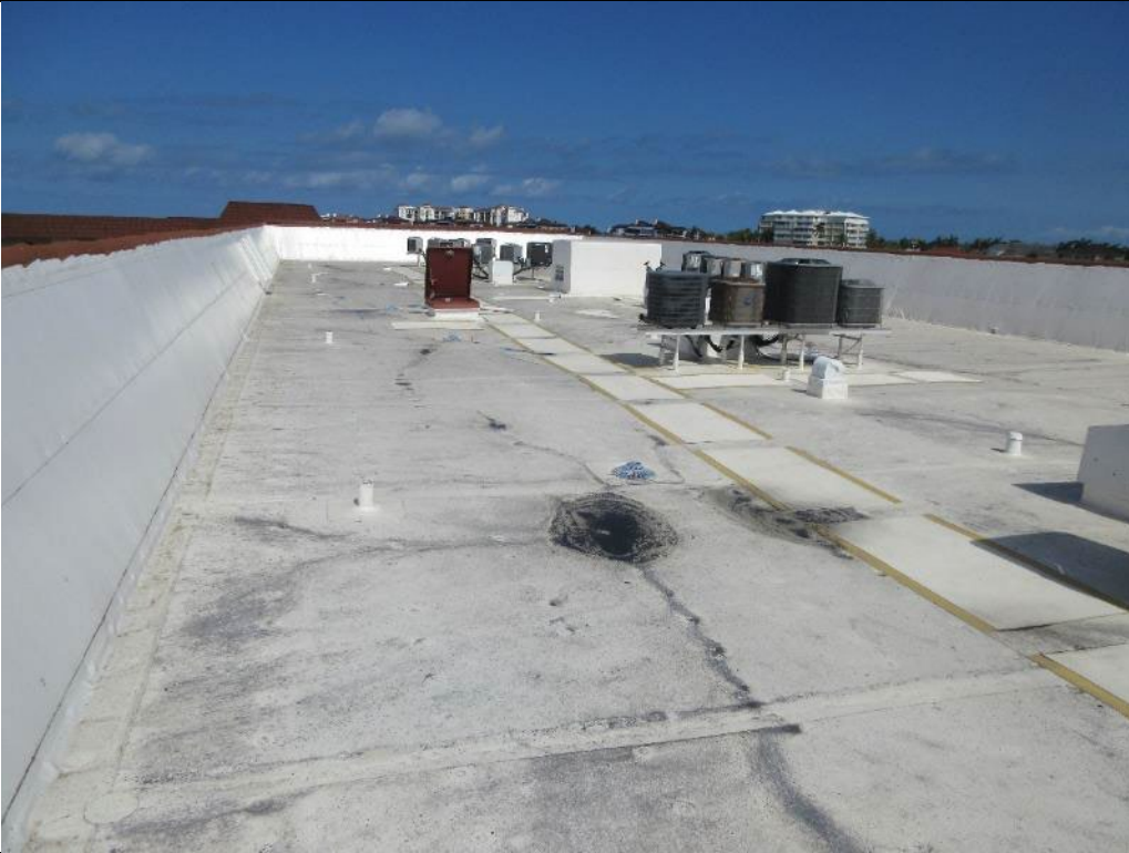
Photo 20. Typical Overview TPO Roof
