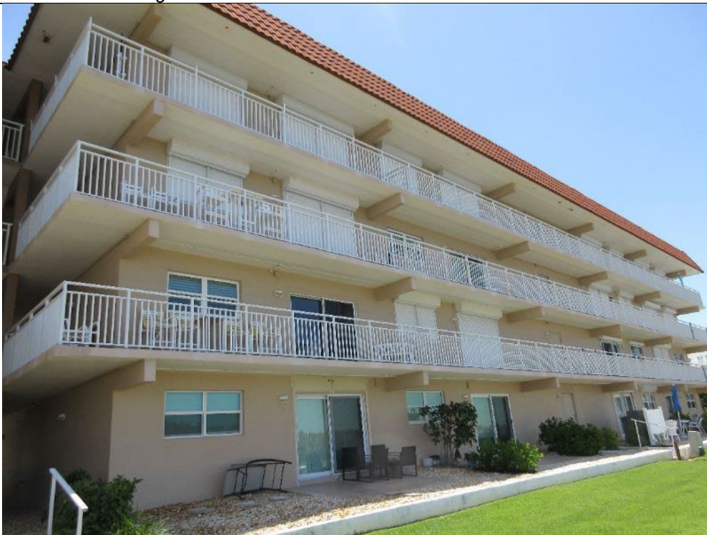
Photo 76. Building E Rear Overview
