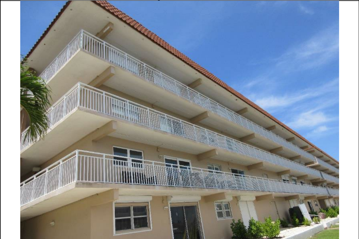
Photo 2. Rear Elevation Building A Overview
