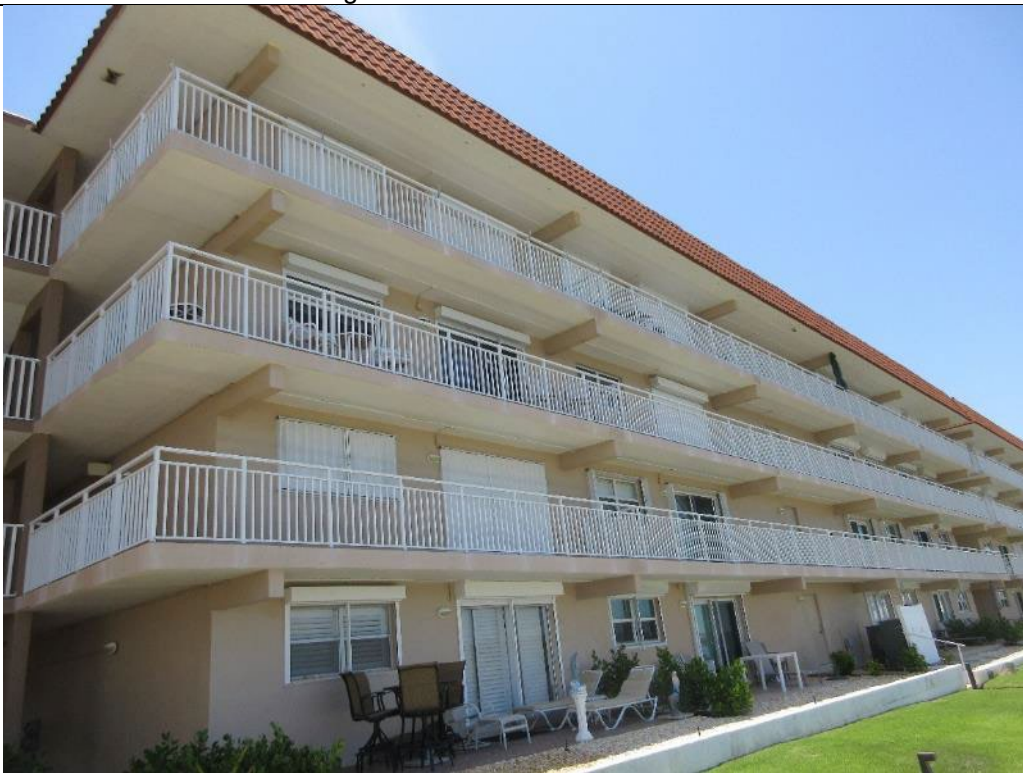
Photo 54. Rear Elevation Building D Overview
