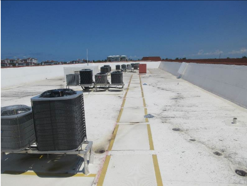
Photo 94. Typical Roof Overview Building E
