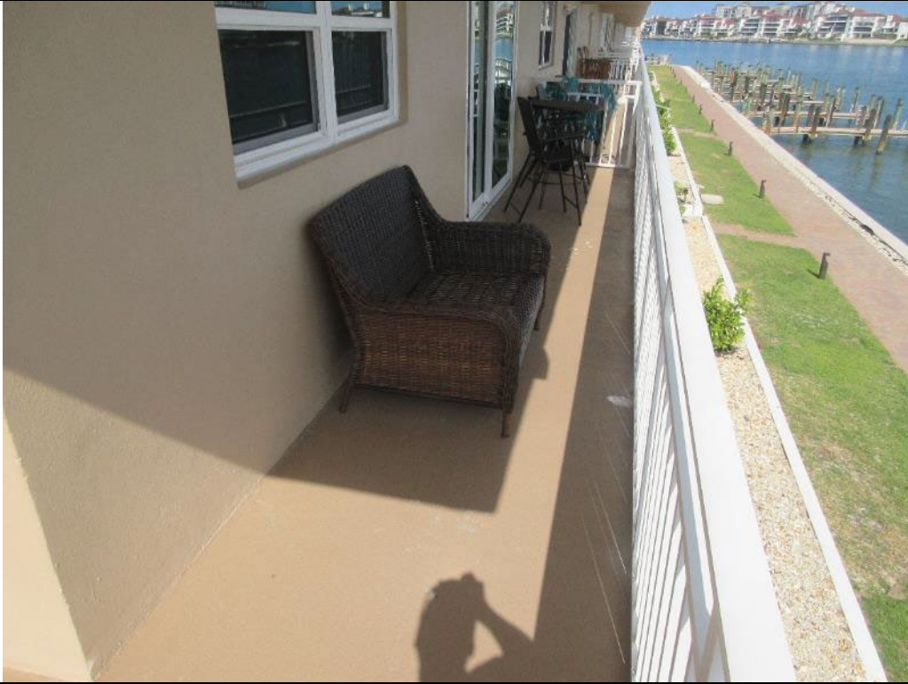
Photo 13. Typical Balcony Overview (Unit A201)
