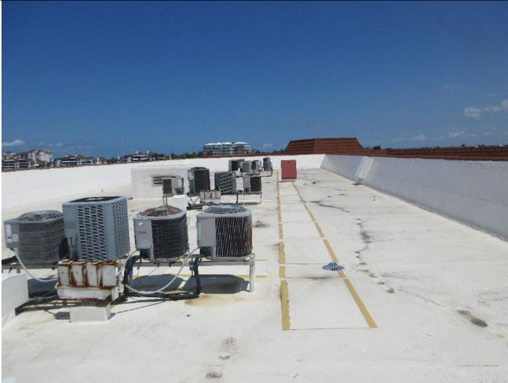
Photo 73. Typical Roof Overview Building S
