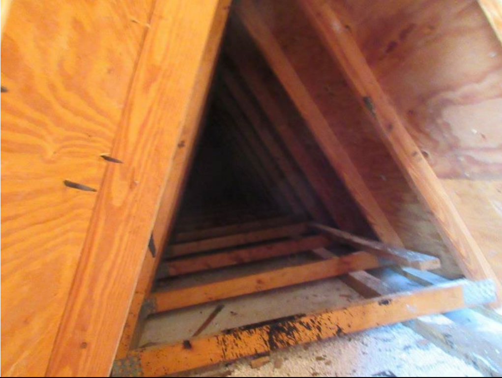
Photo 21. Typical Mansard Roof Trusses
