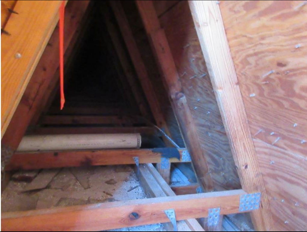
Photo 96. Typical Mansard Truss and Roof Deck Building E
