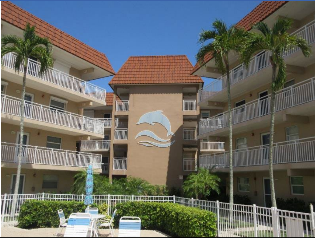
Photo 35. Building C Front Elevation (Building B on Right Building D on Left)
