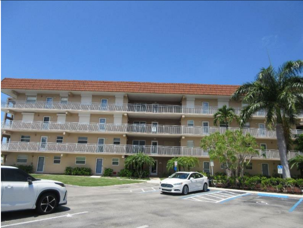
Photo 75. Building E Overview
