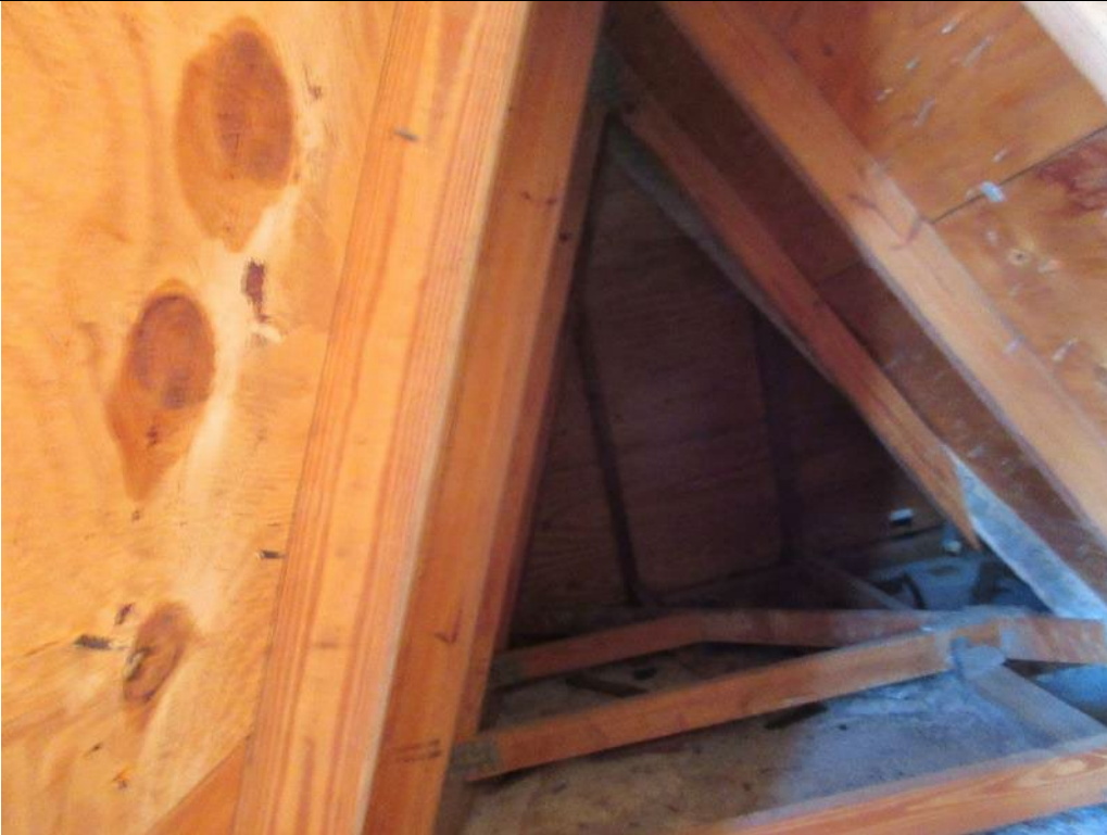
Photo 49. Typical Mansard Roof Trusses
