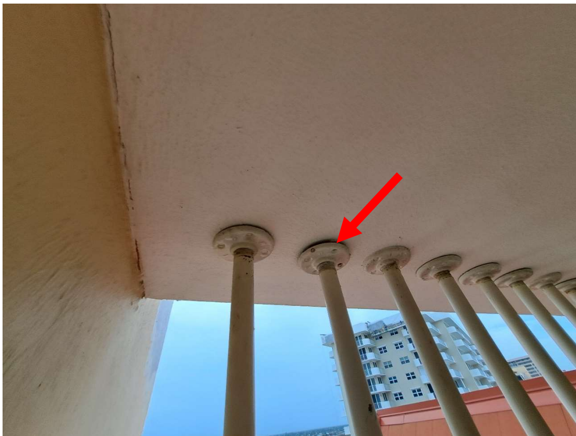
Photo 15 Ref: 2.1.9.1 – Exterior Stair Balcony Barrier Anchors
