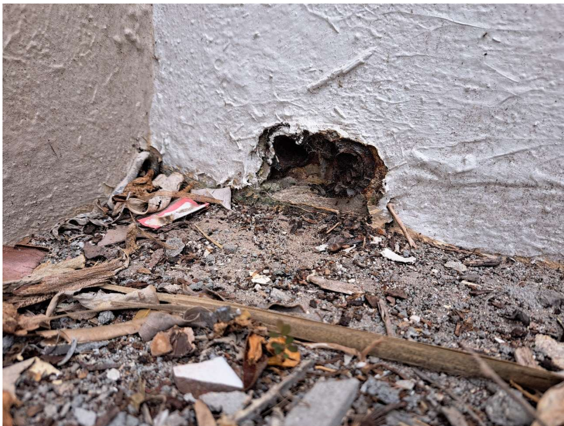
Photo 06 Ref: 2.1.3.1 – Ground-Level Wall Penetration
