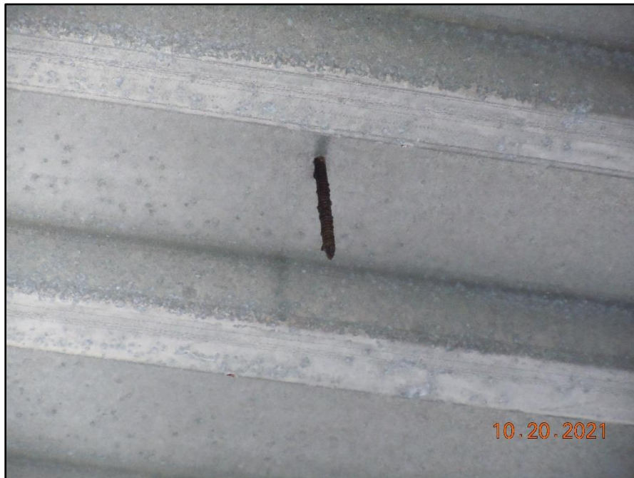
Fastener corrosion
