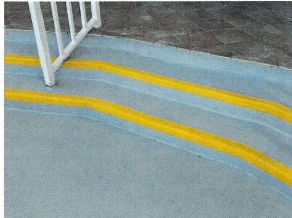
Photo 24: Newly sealed and waterproofed steps to the garage.
