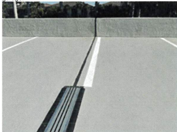
Photo 26: Newly installed expansion joint.
