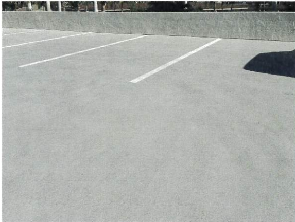
Photo 23: New sealant and waterproofing to the garage.
