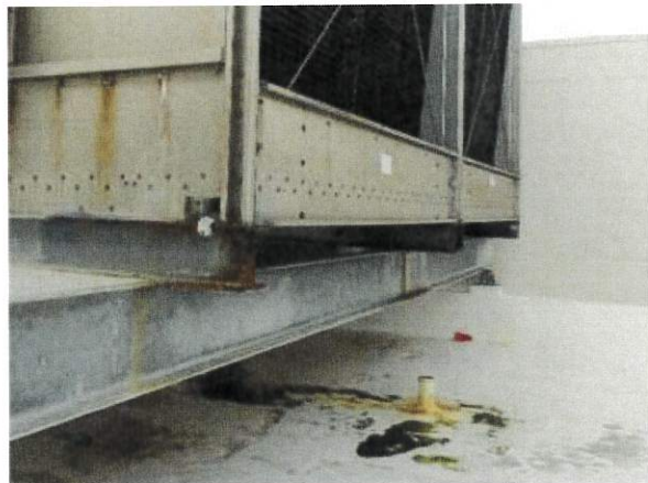
Photo 20: Server corrosion on multiple steel beam.
