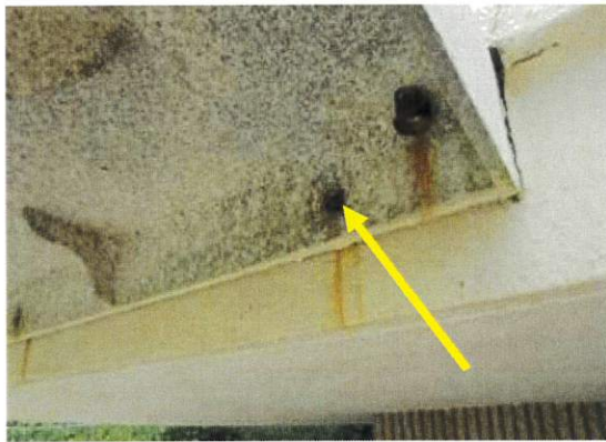
Photo 13: Missing anchor.
