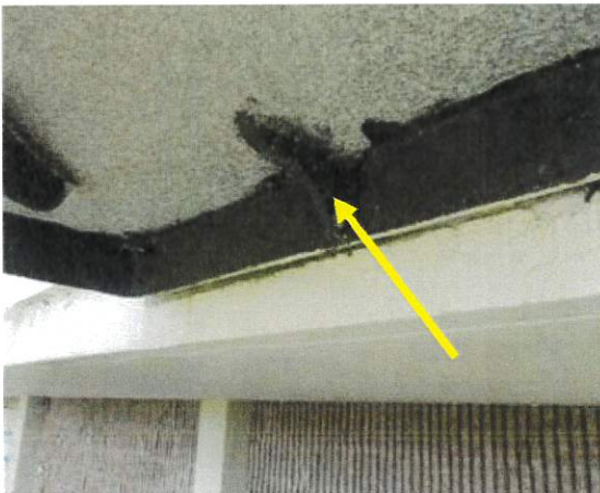
Photo 15: Corroded anchor.
