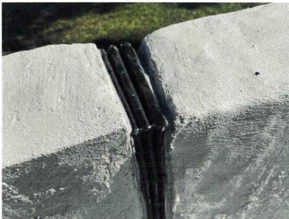
Photo 25: Newly installed expansion joint.
