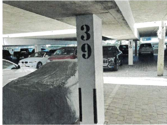
Photo 28: Concrete spalling on column has been repaired.
