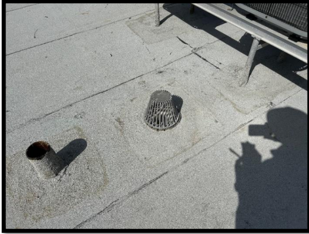
Roof Drains and Scuppers
