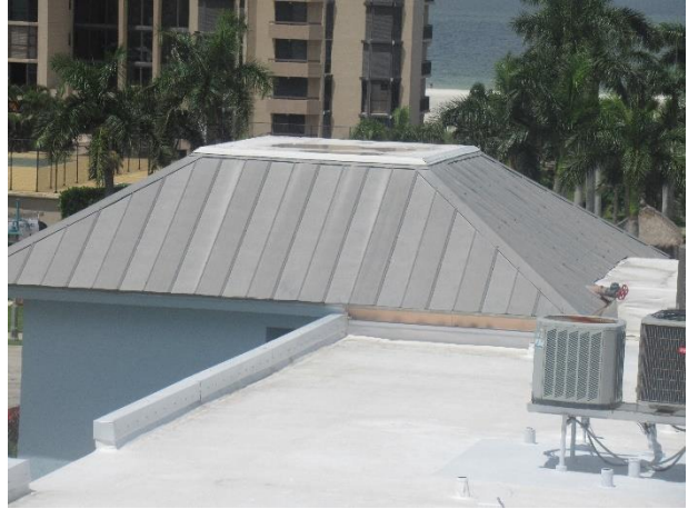
Metal roof overview
