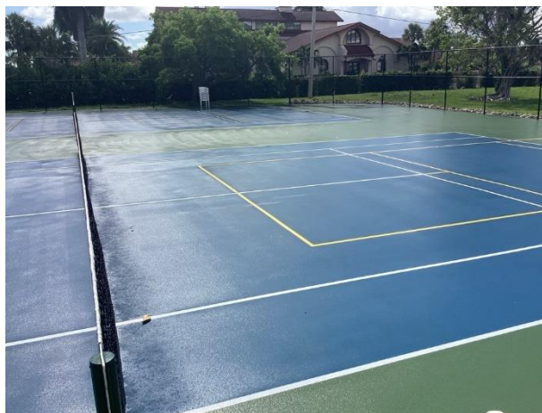
Tennis court overview
