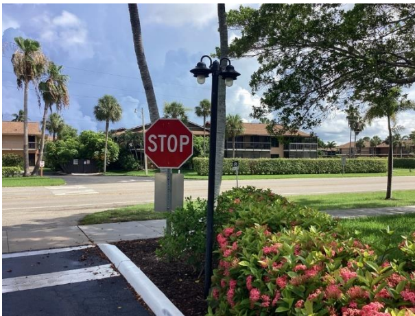
Light pole and fixtures
