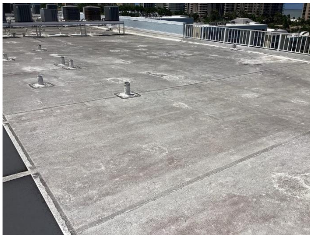
Modified bitumen roof overview – Building C
