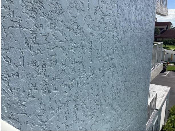
Stucco wall finishes
