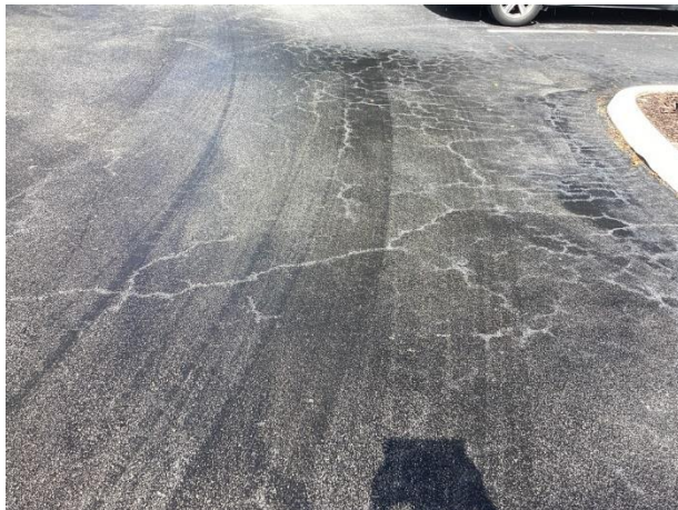
Pavement cracks
