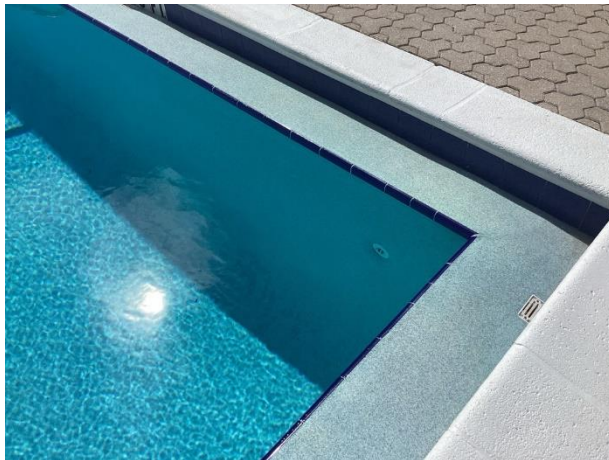
Pool plaster finish with tile perimeter
