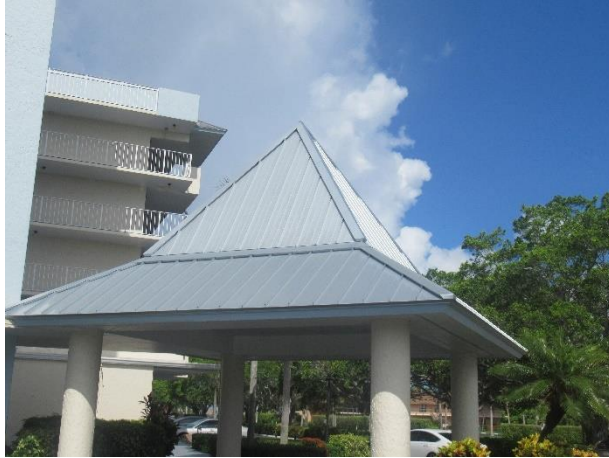
Metal roof overview
