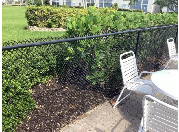
Chain link pool fence
