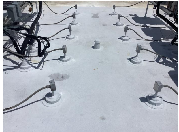
Thermoplastic roof overview
