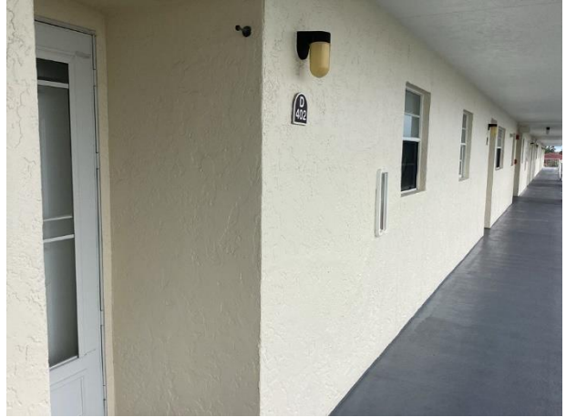
Stucco wall finishes
