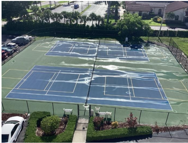
Tennis court overview
