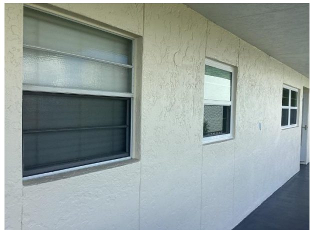
Stucco wall finishes
