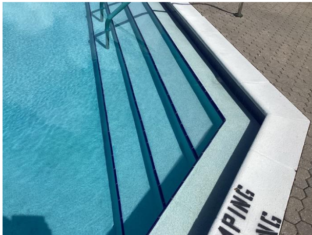
Pool plaster overview
