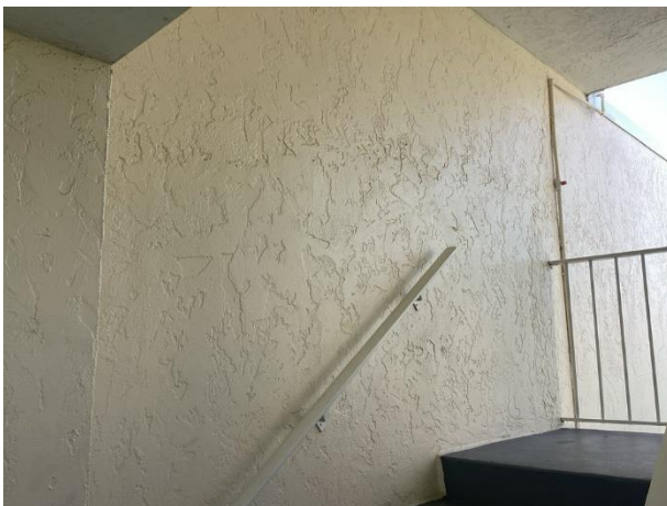
Stucco wall finishes
