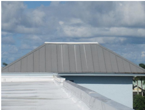
Metal roof overview
