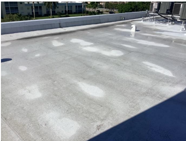
Thermoplastic roof overview
