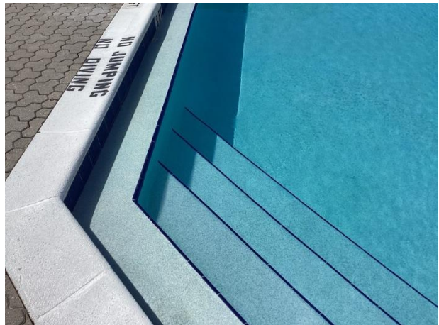
Pool plaster overview
