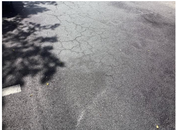
Pavement cracks
