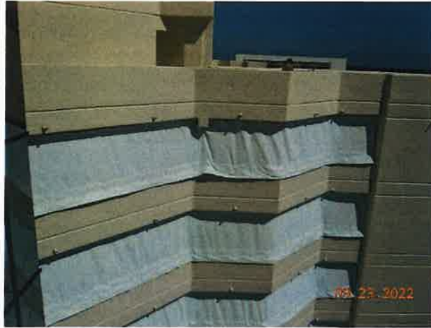
New Hurricane Curtains Being Installed Prior to Hurricane Ian
