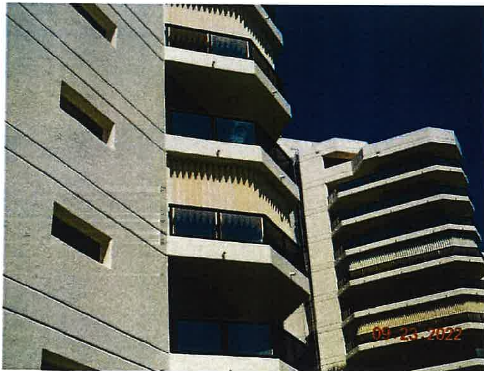
Storm Shutters at Lanais
