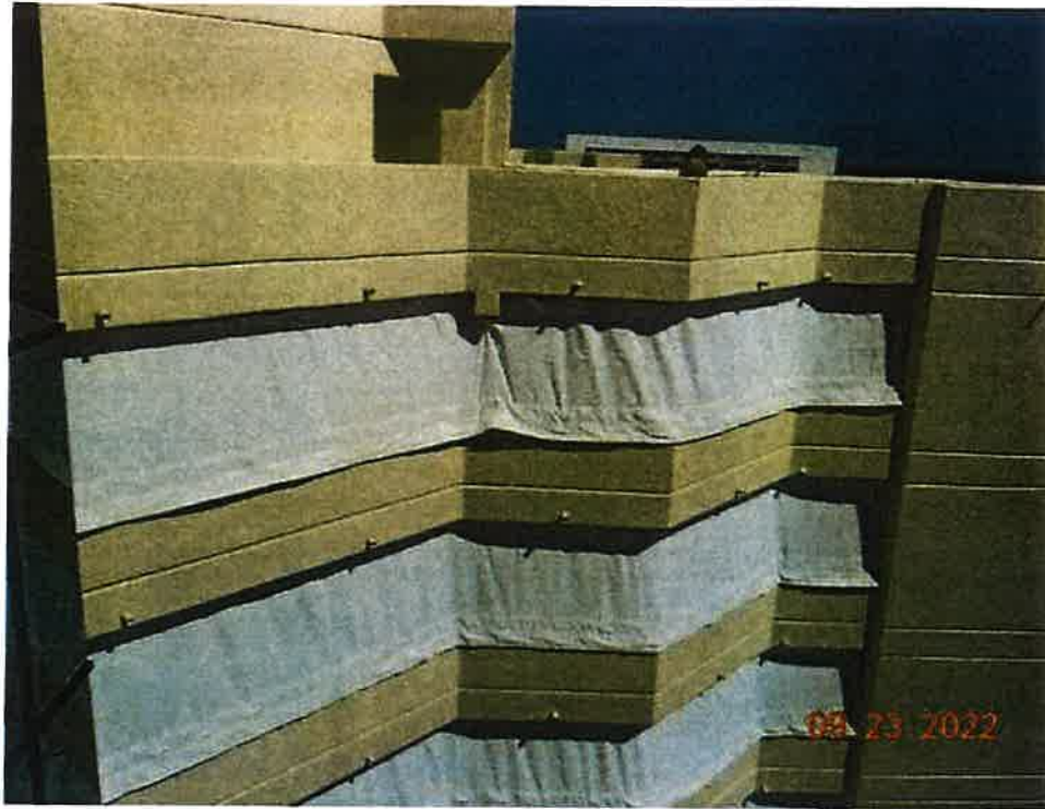
Wind Curtains Being Installed
