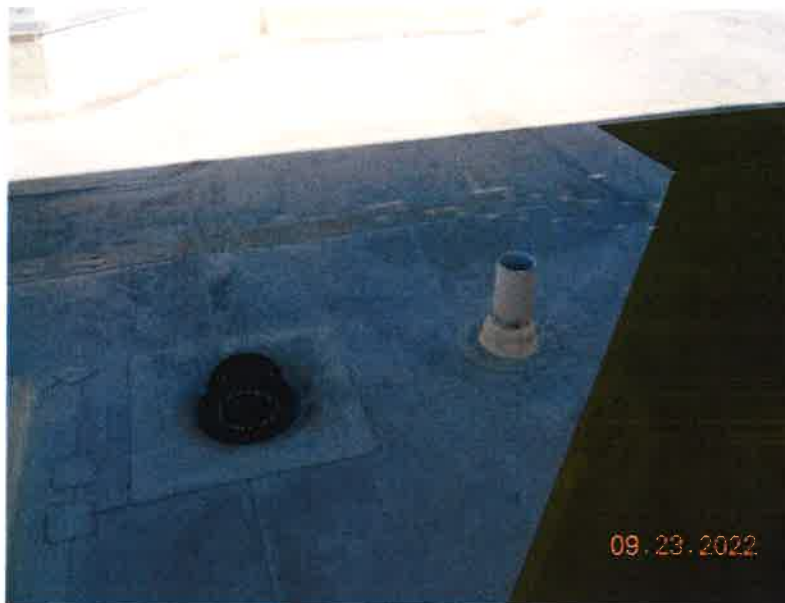
Roof Drain with Overflow
