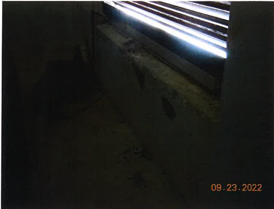
Furnace Roof Louver
