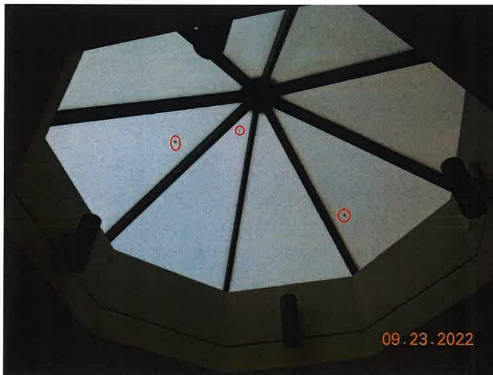
Damaged Skylight
