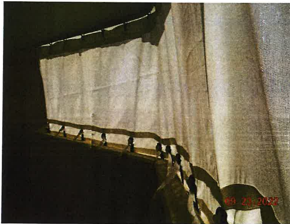
Wind Curtains Being Installed
