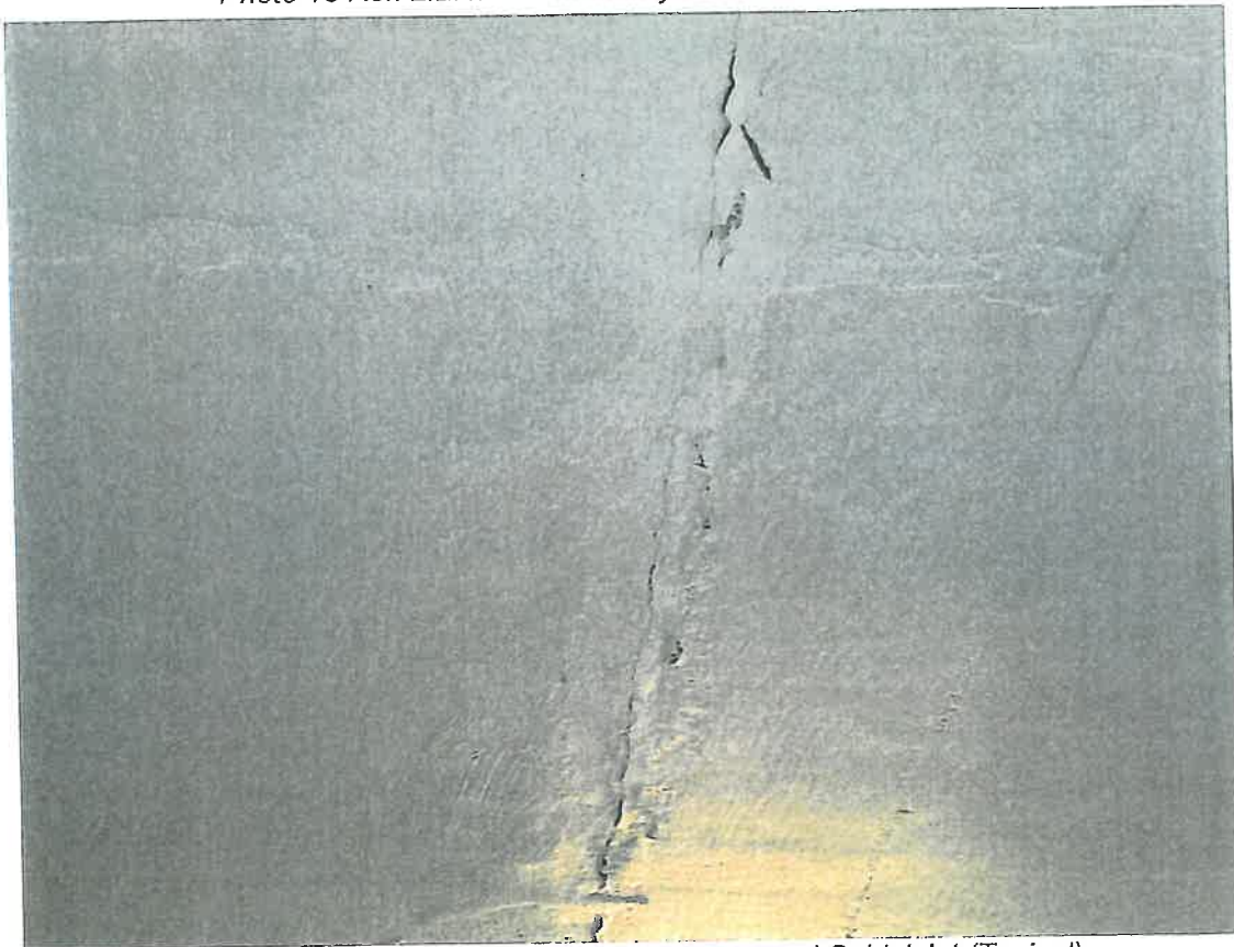
Photo 16 Ref: 2.2.4.1 -- Masonry-Covered Cold Joint (Typical)
