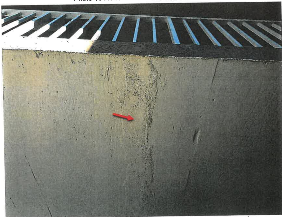
Photo 14 Ref: 2.2.4.1 – Masonry-Covered Cold Joint (Typical)
