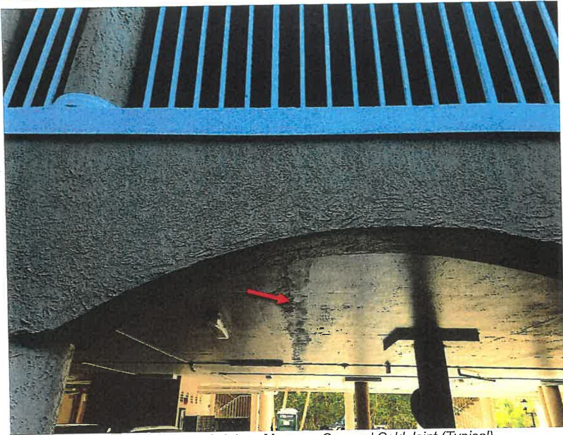
Photo 15 Ref: 2.2.4.1 -- Masonry-Covered Cold Joint (Typical)
