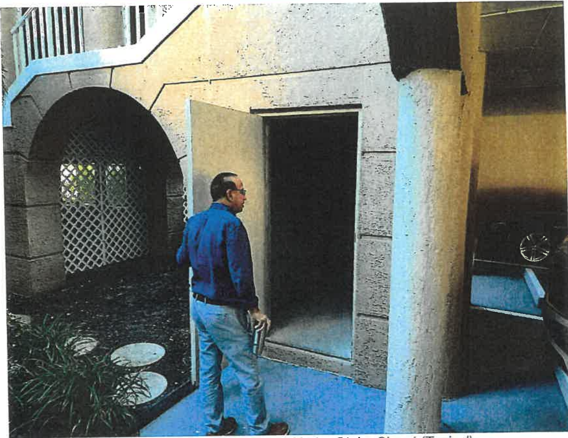
Photo 17 Ref: 2.2.5.1 – Under-Stairs Closet (Typical)
