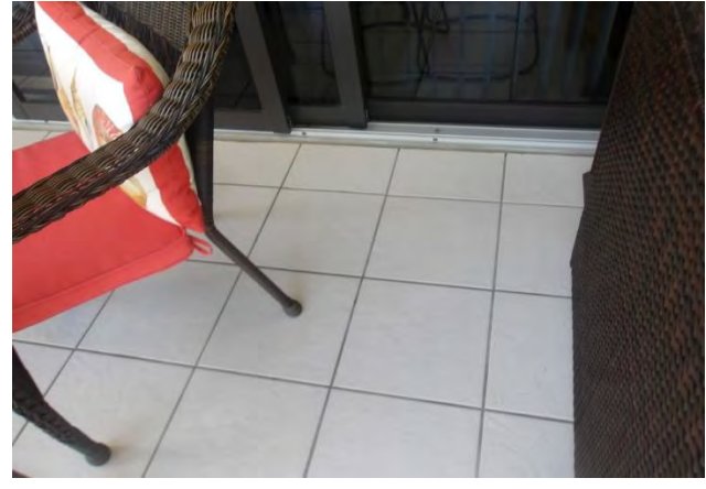
28 Bldg B Balcony Overview Unit #B207
