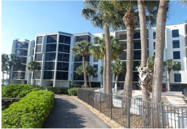
3 Rear of Building B
