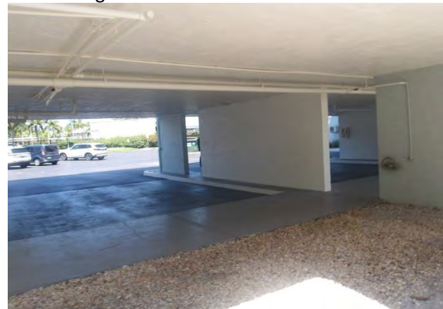
16 Bldg B Pier and Beam Foundation Overview
