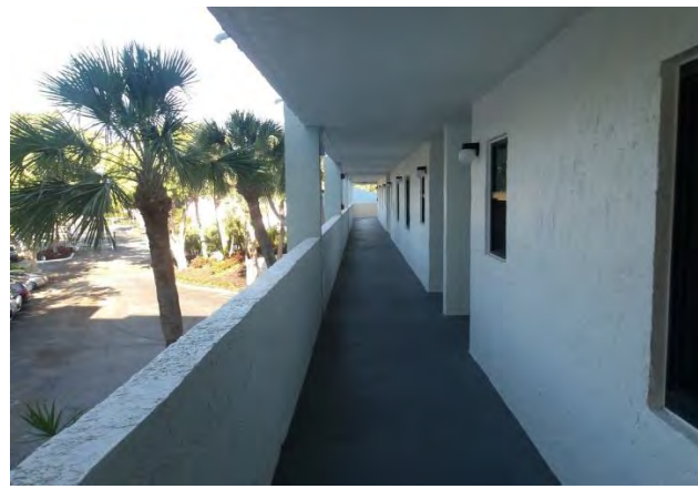
10 Building B Exterior Walls and Breezeways
