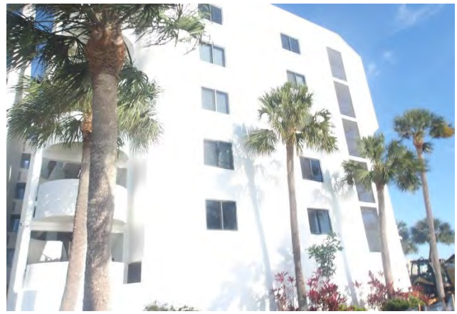
2 Right Side of Building B
