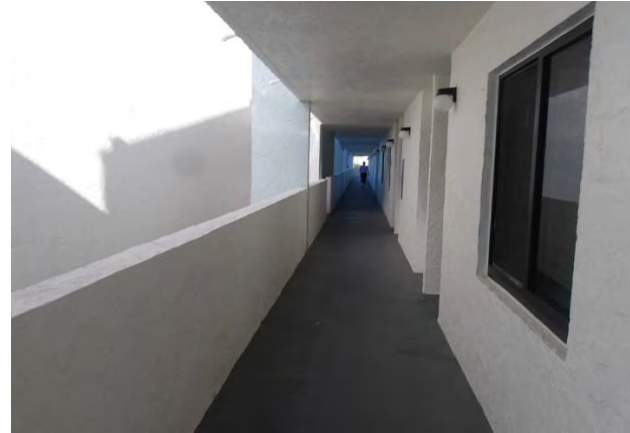
12 Building B Exterior Walls and Breezeways
