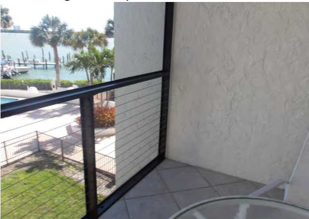
23 Bldg B Balcony Overview Unit #B308
