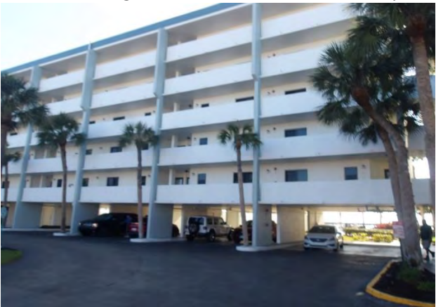
13 Bldg B Pier and Beam Foundation Overview
