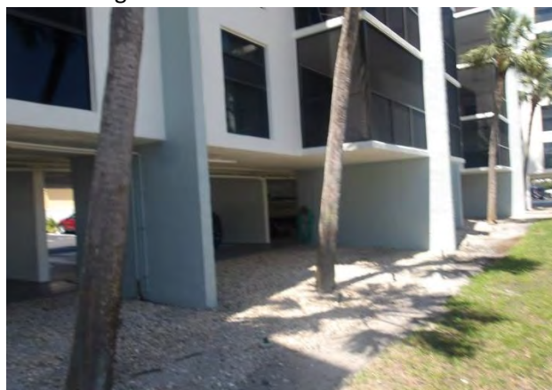
15 Bldg B Pier and Beam Foundation Overview
