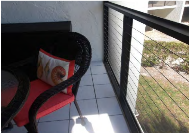
27 Bldg B Balcony Overview Unit #B207
