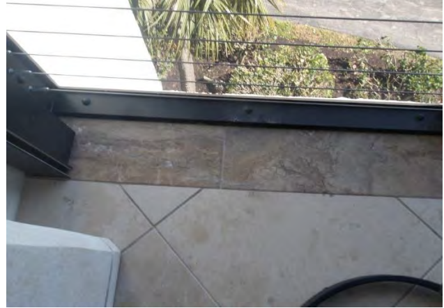
22 Bldg B Balcony Overview Unit #B402
