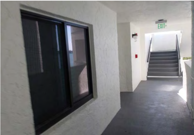
11 Building B Exterior Walls and Breezeways
