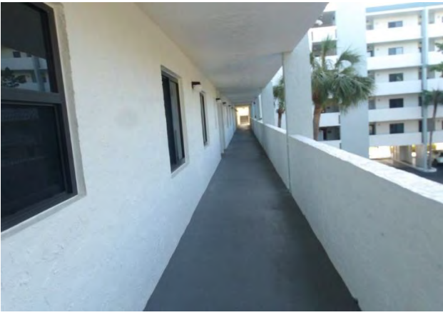
9 Building B Exterior Walls and Breezeways
