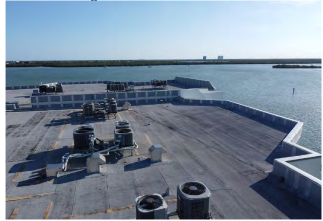
8 Building B Roof Overview
