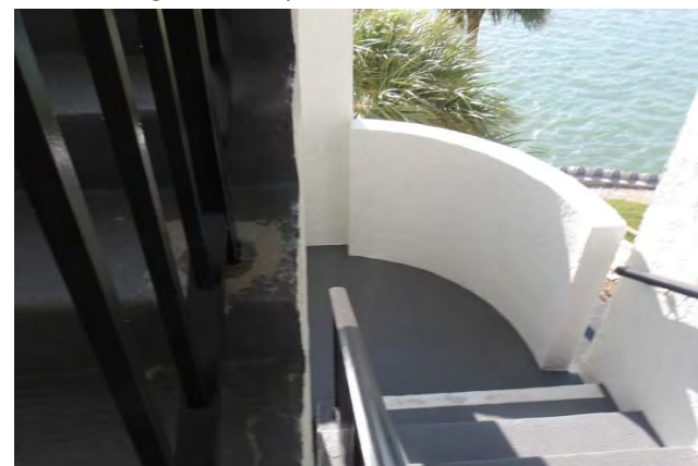
30 Bldg. B Stairway Overview
