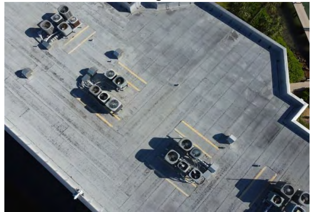
6 Building B Roof Overview
