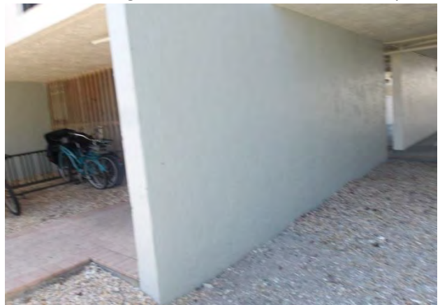
14 Bldg B Pier and Beam Foundation Overview
