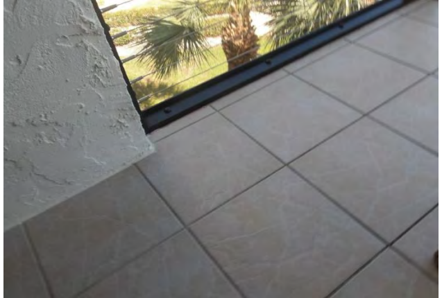
20 Bldg B Balcony Overview Unit #B406
