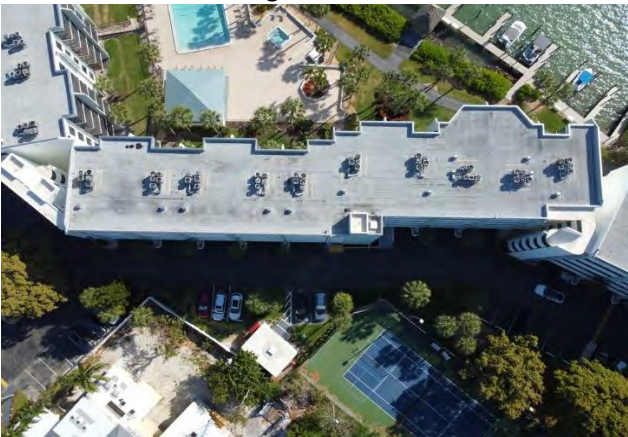
5 Building B Roof Overview
