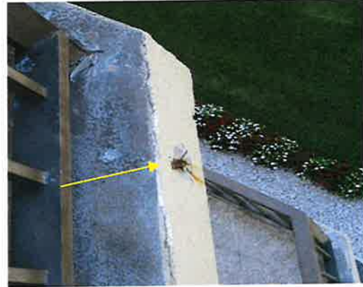
View of exposed and corroded steel reinforcement along deck edge.
