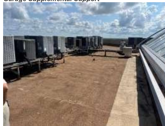
Roof overall condition.
