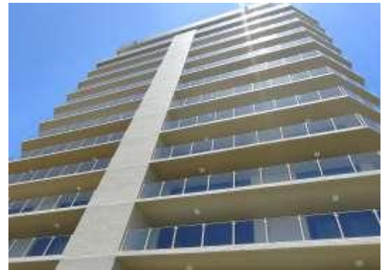
Exterior of the structure.
