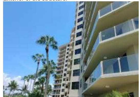
Exterior of the structure
