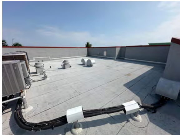
VIEW OF ROOF TOP
