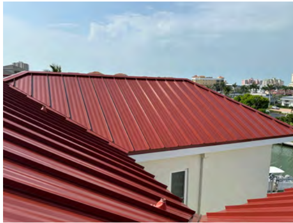
VIEW OF MANSARD COVERINGS
