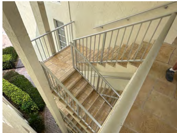
VIEW OF TYPICAL STAIR SYSTEM
