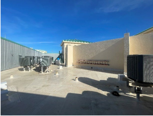
View on top of roof.
