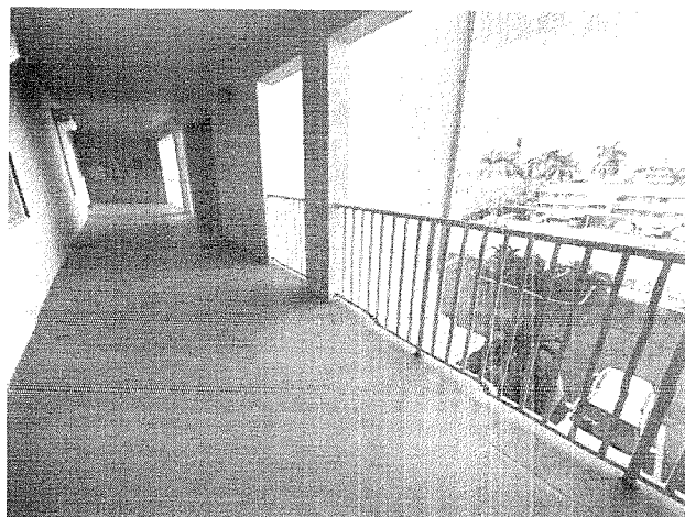
GENERAL VIEW OF TYPICAL ELEVATED WALKWAY
