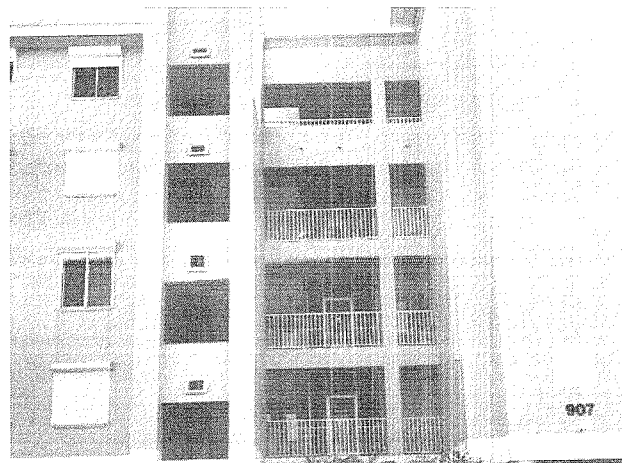
GENERAL VIEW OF GUARDRAILS
