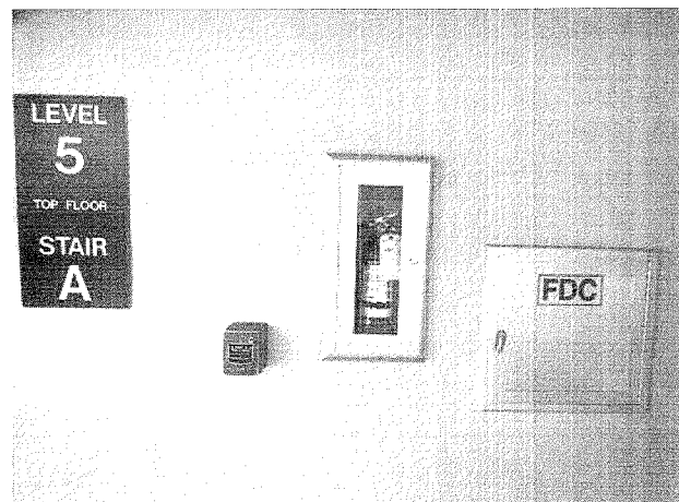
GENERAL VIEW OF FIRE EXTINGUISHER
