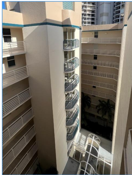
Figure 8: Exterior catwalks and Non-Accessible Juliet Balconies
