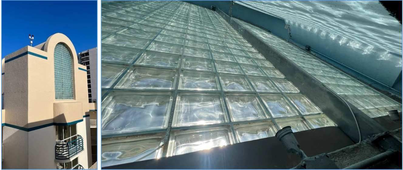
Figure 19: Rooftop glass enclosure
