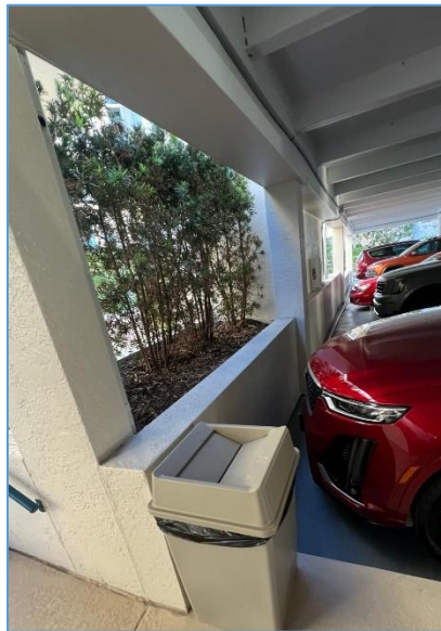
Figure 10: Planter and square column cover to be investigated at west side of garage
