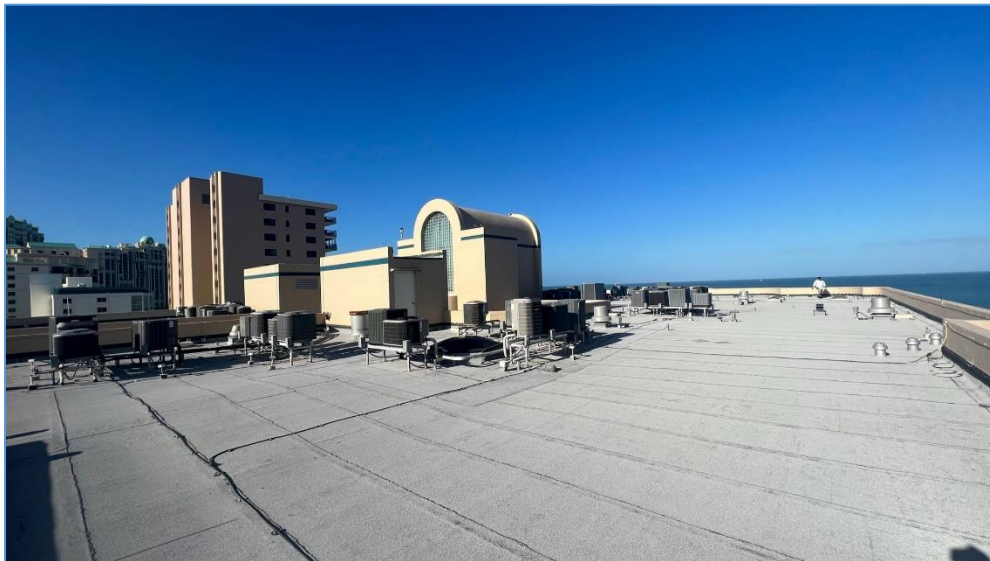
Figure 16: Main building roof
