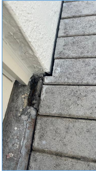
Figure 6: Reinforced concrete repair at entrance of Cabana 9
