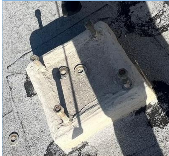
Figure 17: Typical roof anchor system
