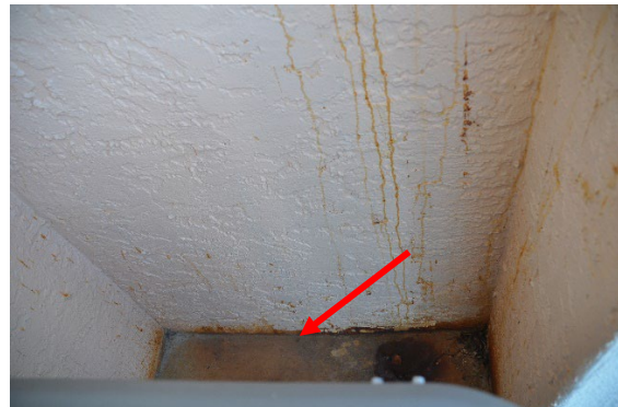
20. Exposed rogue piece of steel reinforcement. Too little coverage was provided during construction in service area 402
