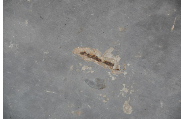
20. Exposed rogue piece of steel reinforcement. Too little coverage was provided during construction in service area 402
