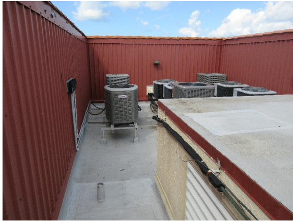
Typical Condo Modified Bituminous Roof
