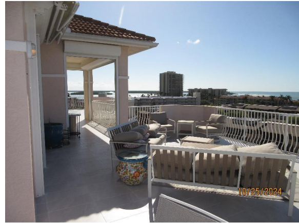
Typical Penthouse Level Railings
