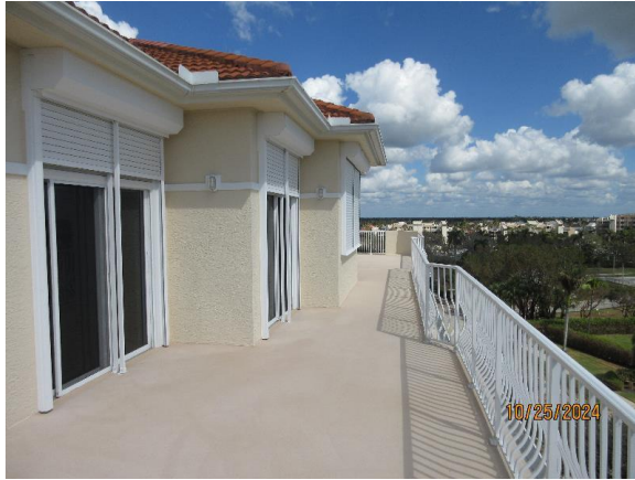
Typical Penthouse Level Railings
