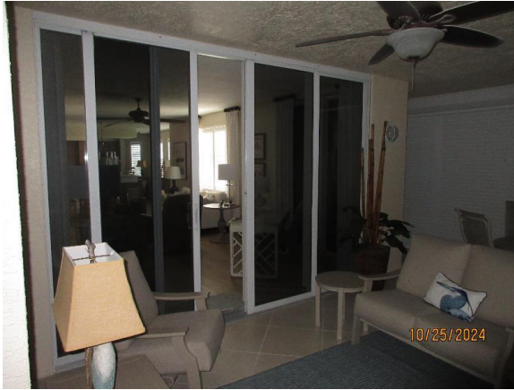
Typical Rear Balcony Sliding Glass Door
