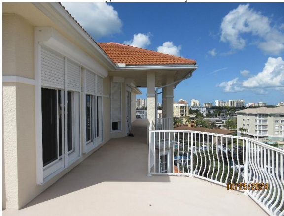
Penthouse Balcony Deck Over Occupied Space
