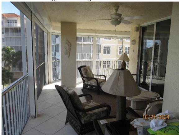
Typical Rear Balcony Overview and Column
