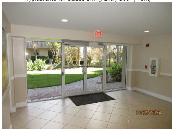
Typical Rear Storefront Door and Window System
