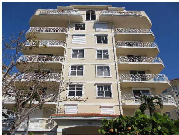
Typical Overview Front Balcony Aluminum Railings
