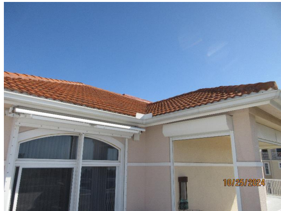
Close-Up Roof Overview
