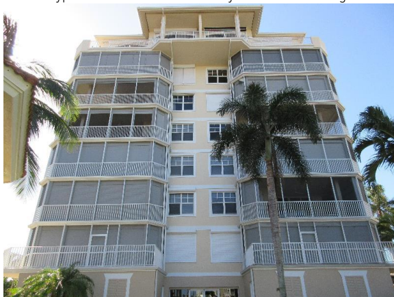
Typical Overview Rear Balcony Enclosure with Integral Railings
