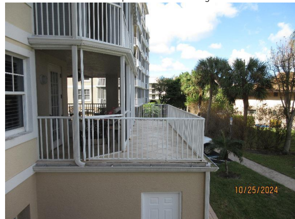
2 nd Level Balcony Railings and Enclosure
