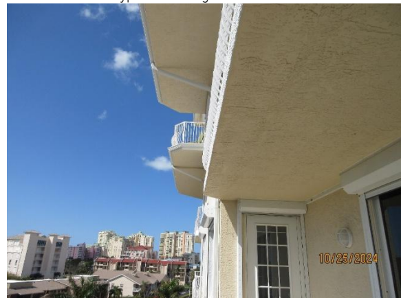
Front Balcony Ceiling and Slab
