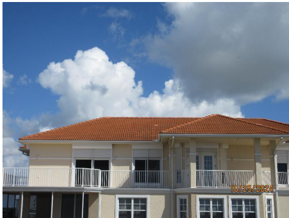
Typical Roof Overview
