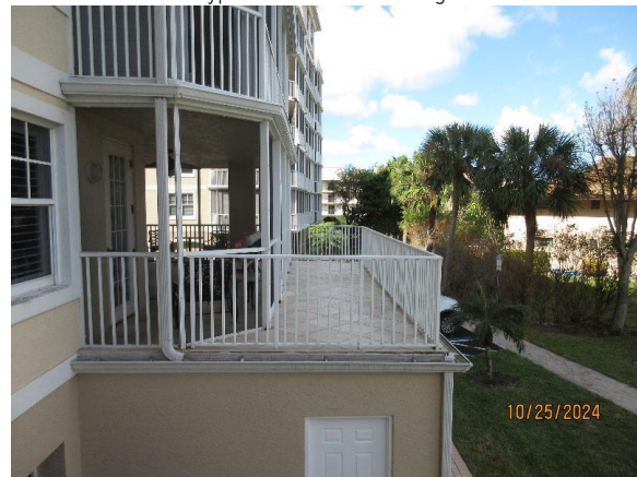
2 nd Level Balcony Deck Over Occupied Space
