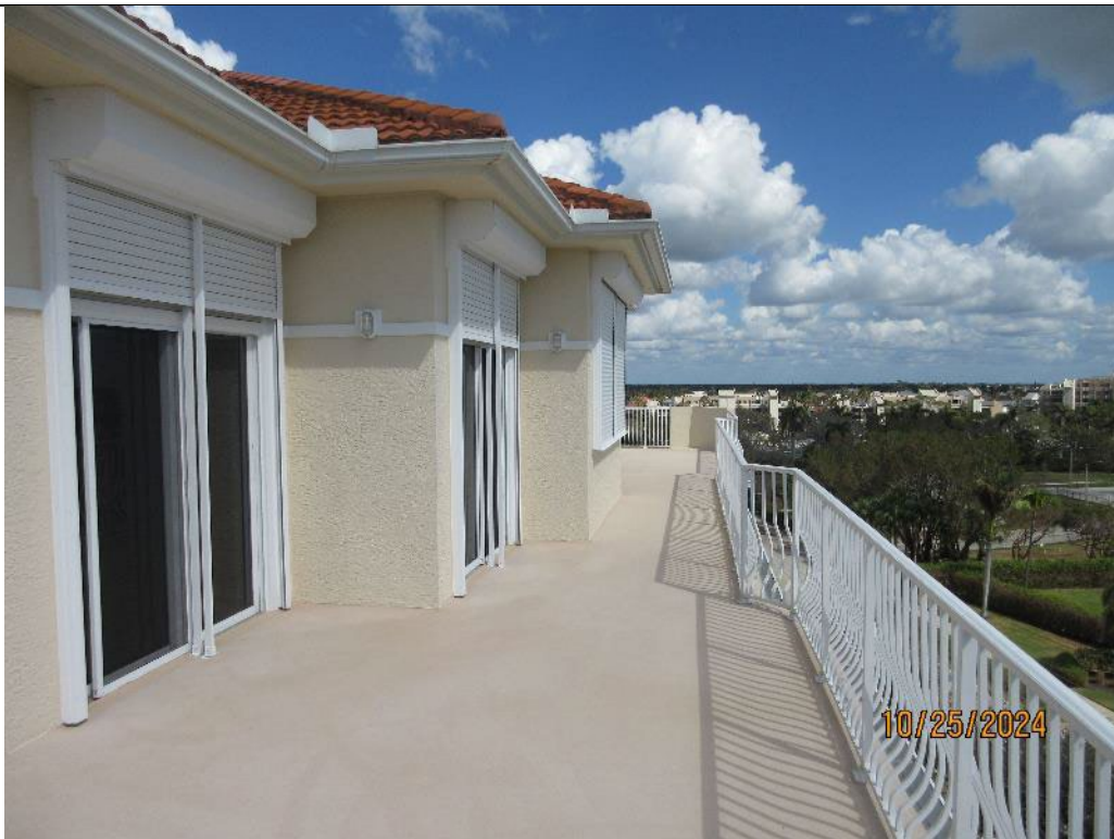
Photo 18. Overview Typical Penthouse Wrap Around Balcony
