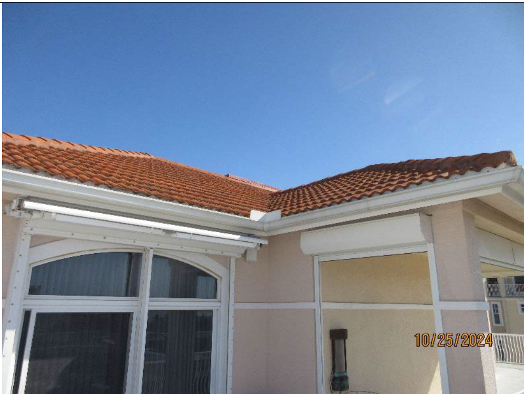
Photo 32. Close Up Concrete Tile Roof
