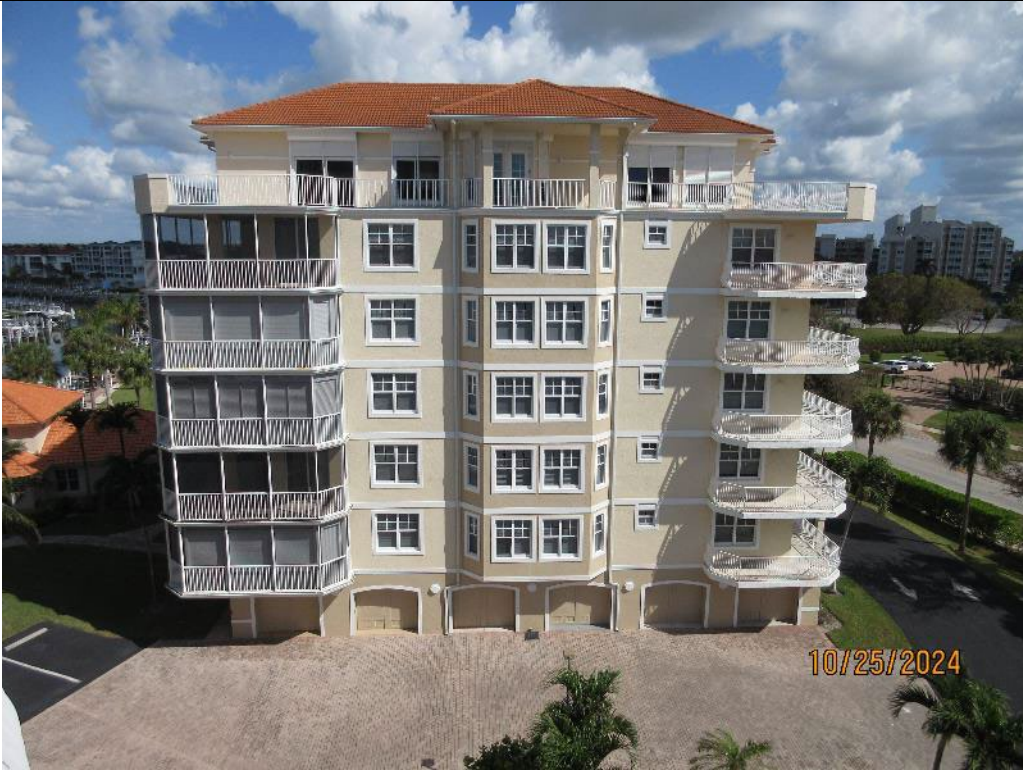
Photo 3. Similar Side Elevation of Seven-Story Building
