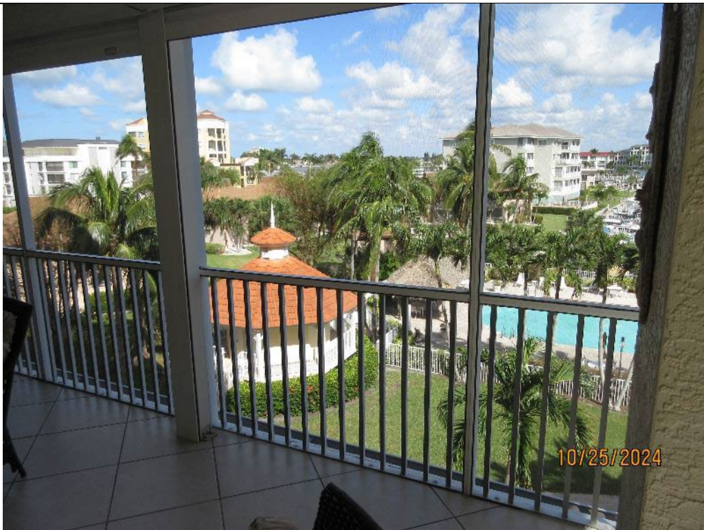
Photo 14. Typical Rear Balcony Screen Enclosure with Integral Guard Railings
