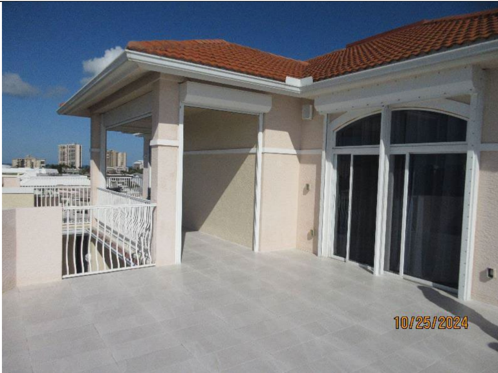
Photo 20. Overview Typical Penthouse Wrap Around Balcony
