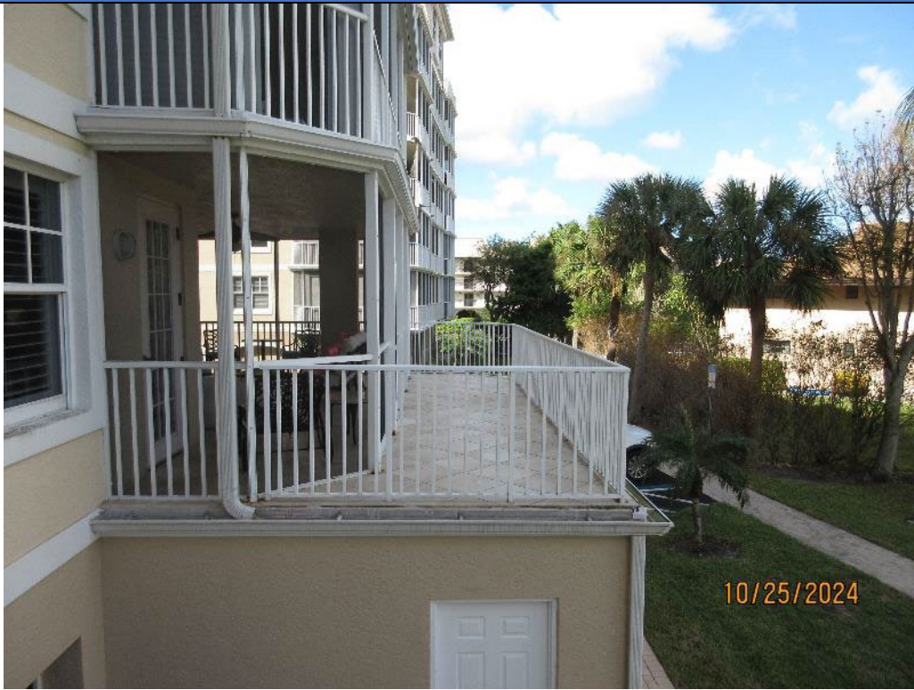
Photo 23. 2 nd Floor Balcony Over Occupied Space
