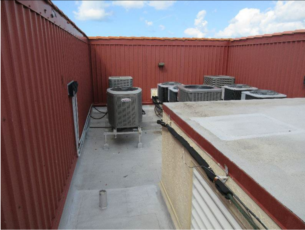
Photo 33. Typical Modified Bituminous Roof System Overview and Mansard Fascia Wall
