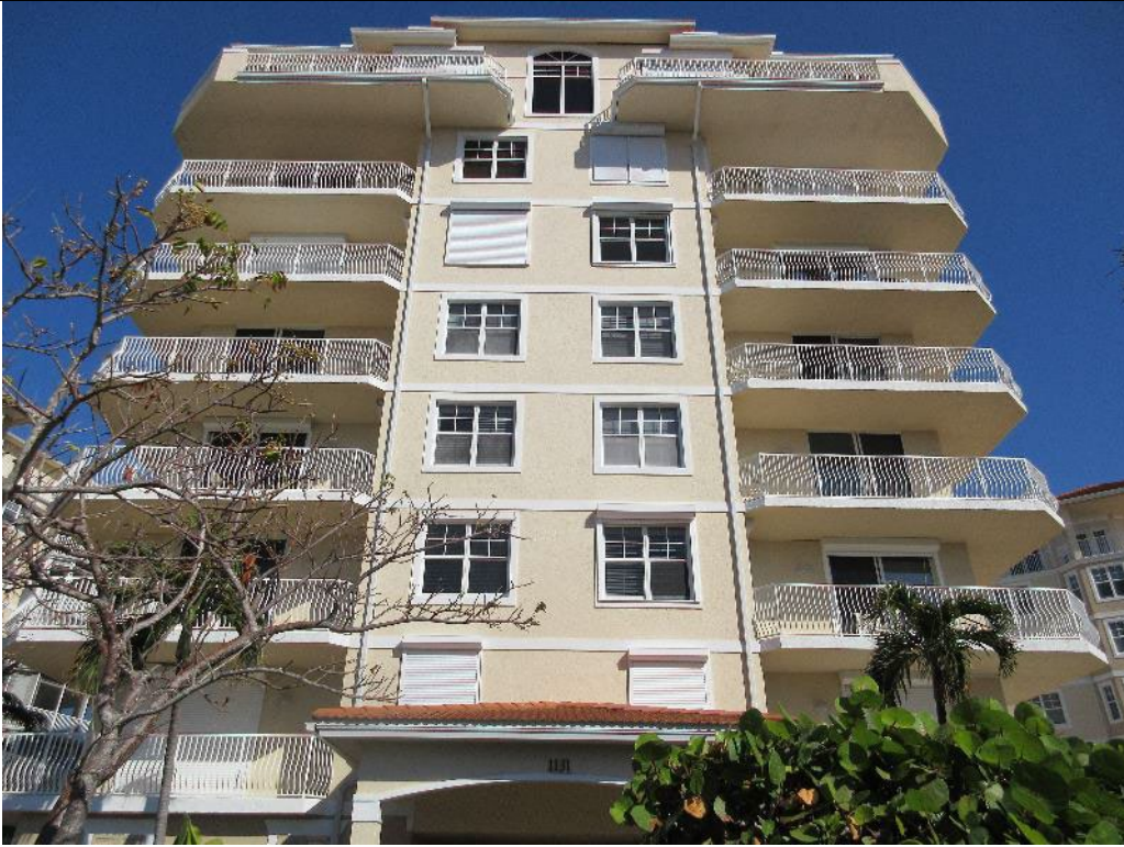
Photo 1. Similar Front Elevation of Each Building
