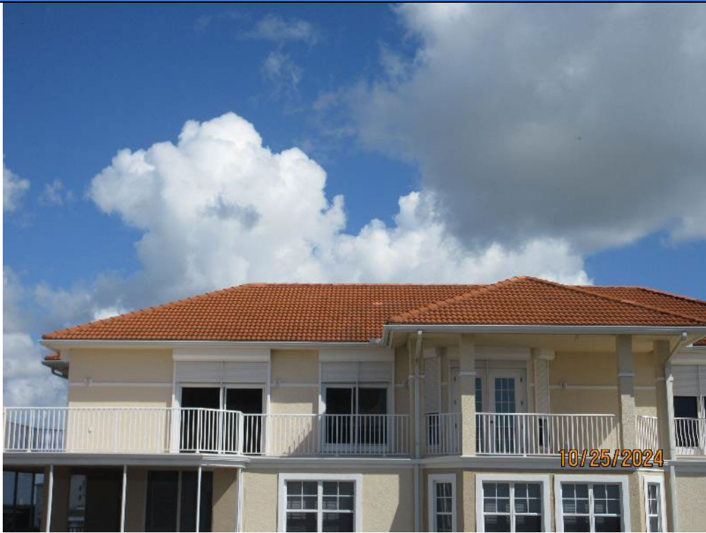
Photo 31. Overview Typical Concrete Tile Roof
