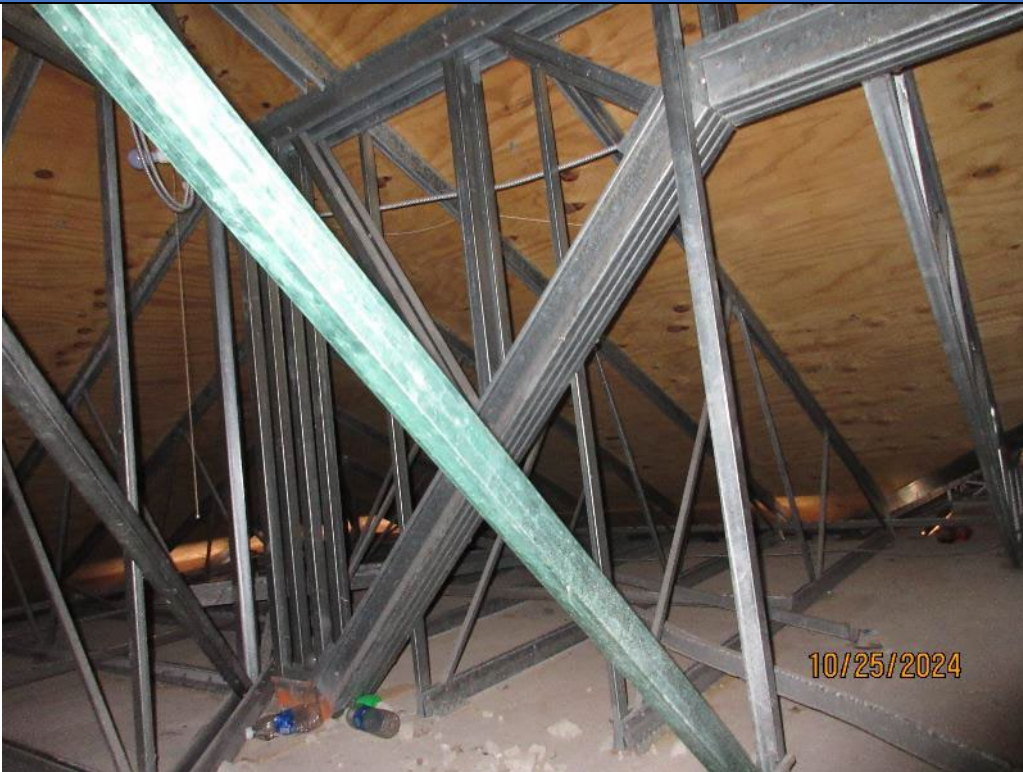
Photo 35. Typical Overview Concrete Tile Roof Truss Framing and Plywood Decking
