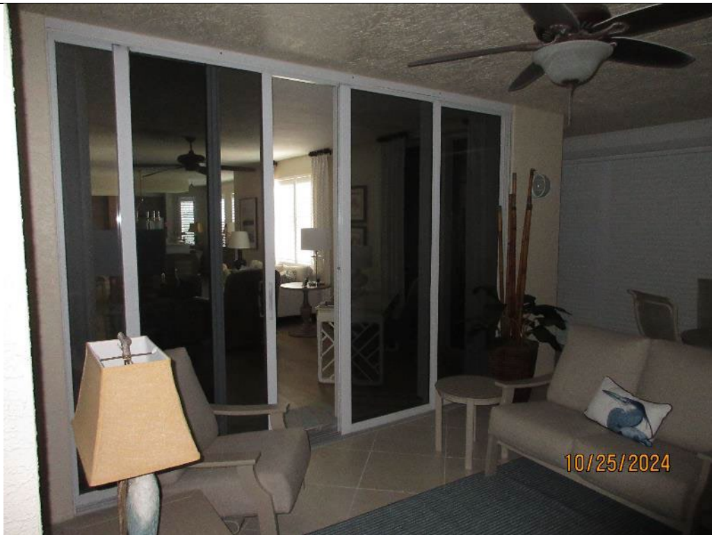
Photo 16. Typical Unit Rear Balcony Sliding Glass Door
