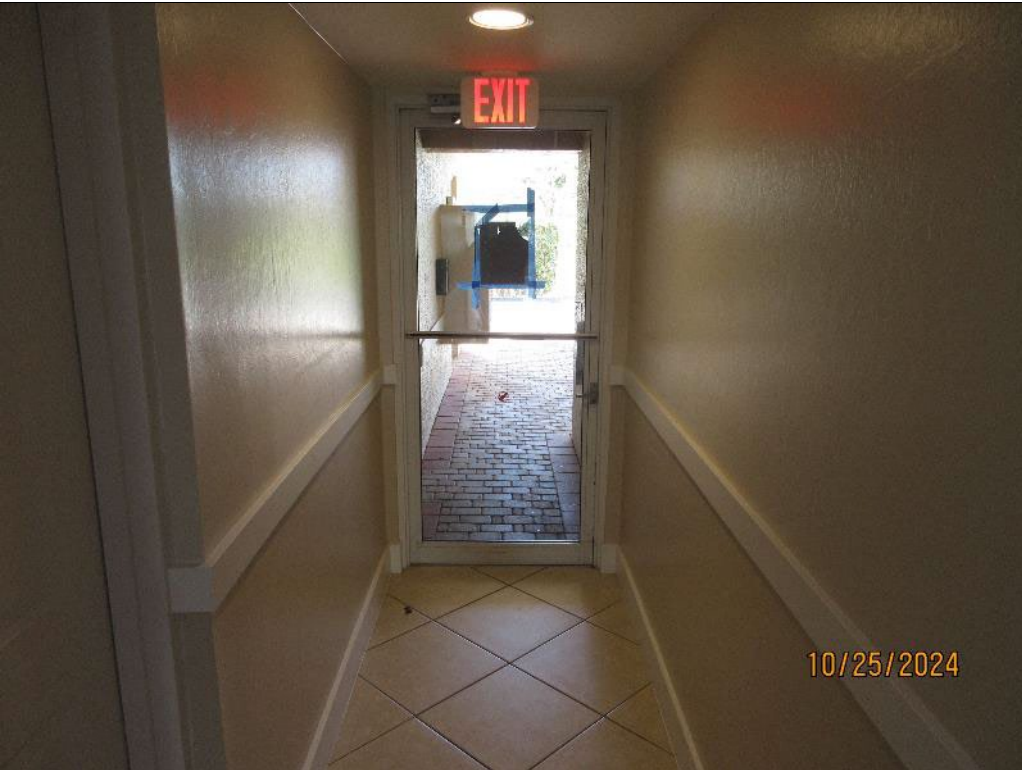
Photo 6. Typical Front Single Glazed Swing Door
