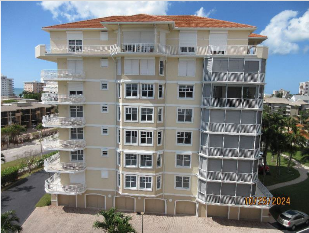
Photo 4. Similar Side Elevation of Eight-Story Building
