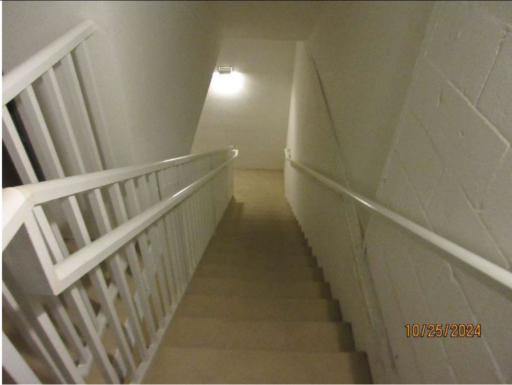
Photo 9. Typical Interior Stair Tower Railings
