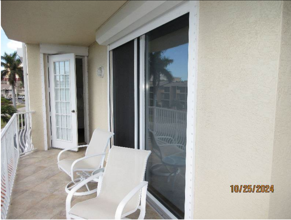
Photo 11. Typical Unit Front Balcony Doors
