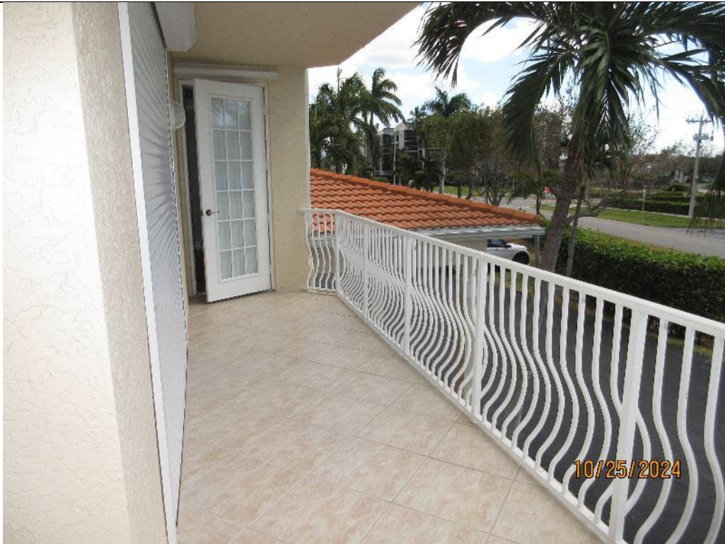
Photo 10. Overview Typical Unit Front Balcony and Railings Overview
