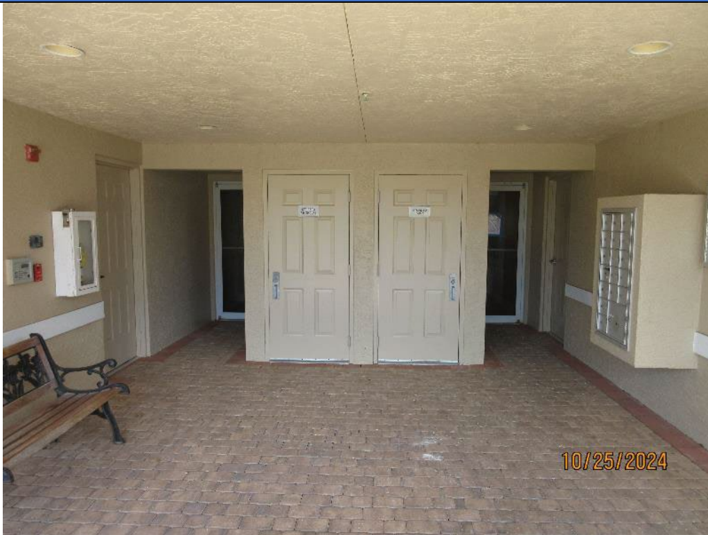
Photo 5. Typical Building Front Entrance and Doors to Internal Stair Towers
