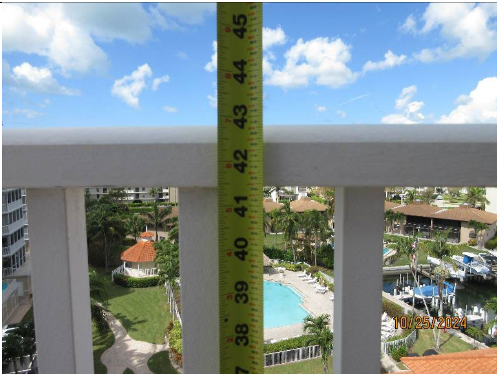
Photo 24. Typical Measured Railing Height > 42"
