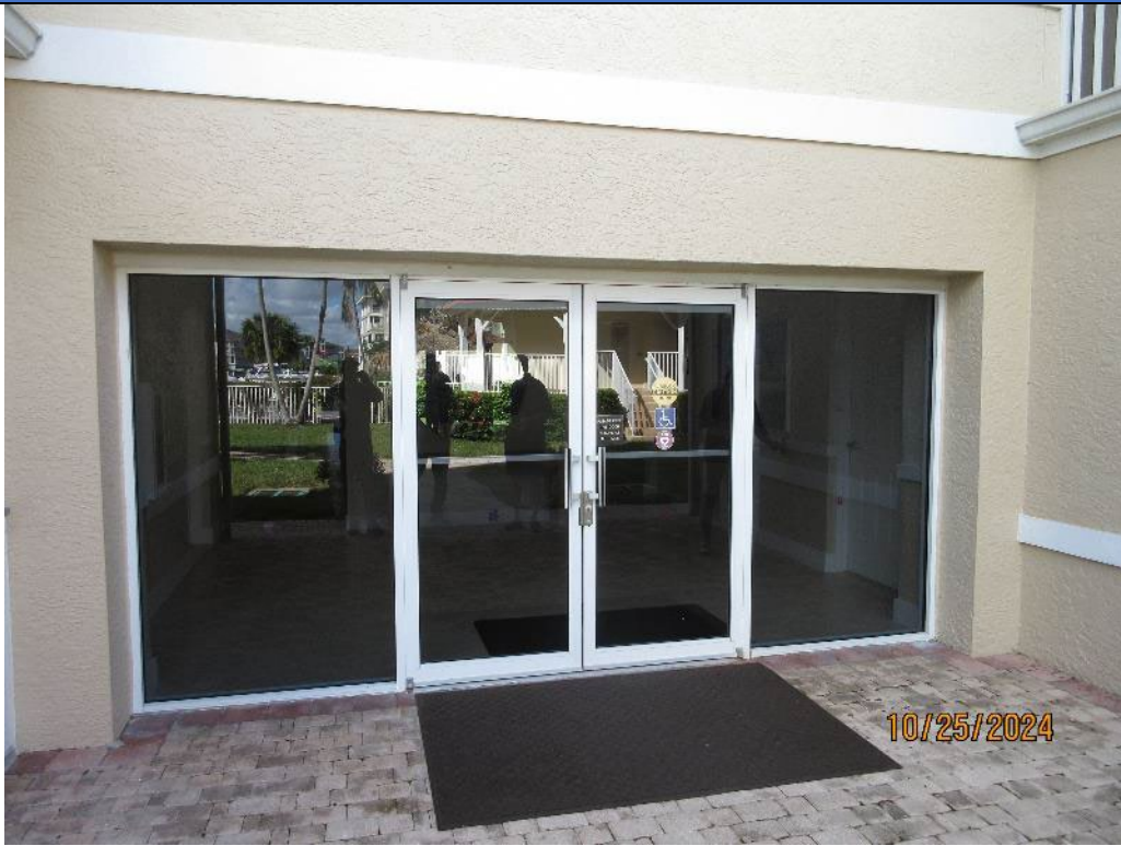
Photo 7. Typical Building Rear Entrance Storefront Door and Window System
