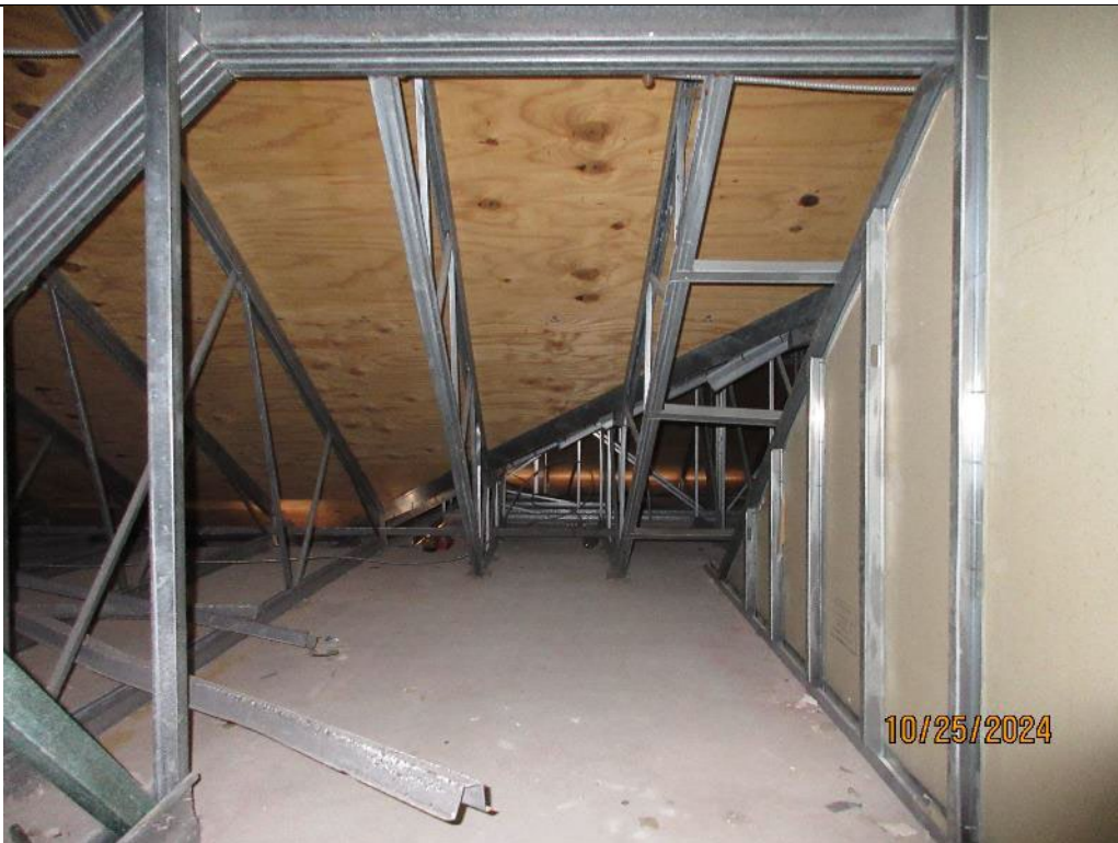
Photo 34. Typical Overview Concrete Tile Roof Truss Framing and Plywood Decking
