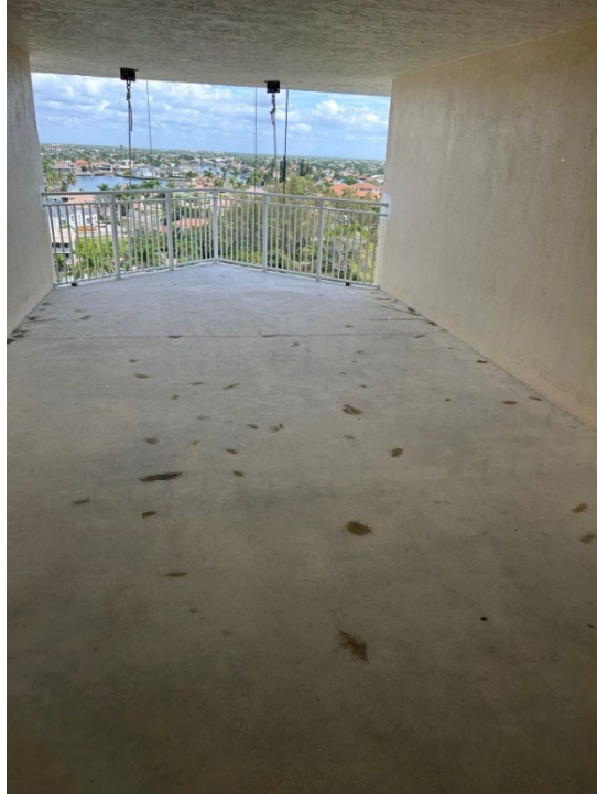
11. View of the concrete repairs being performed on the exterior of the building.
