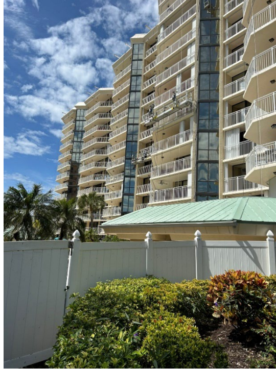
7. View of the repairs being performed on the exteriors and balconies.
