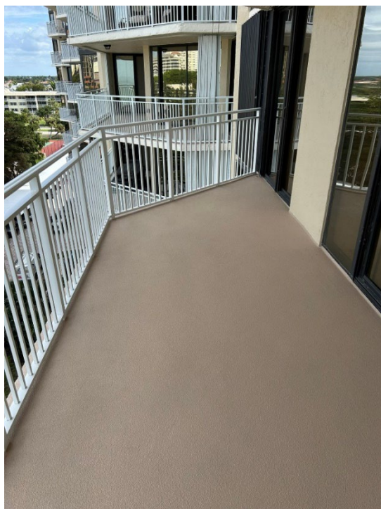
10. View of the balconies being recoated.
