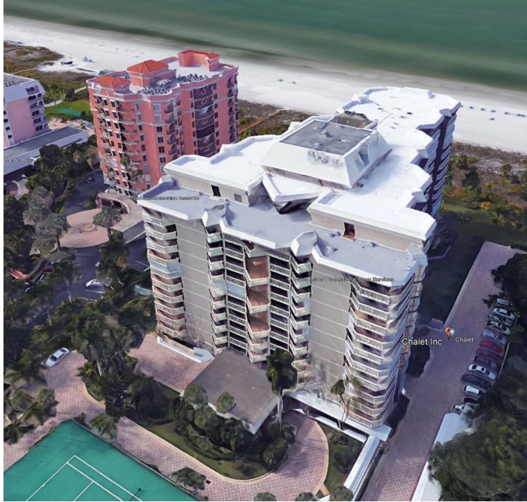
1. View of the subject building.
