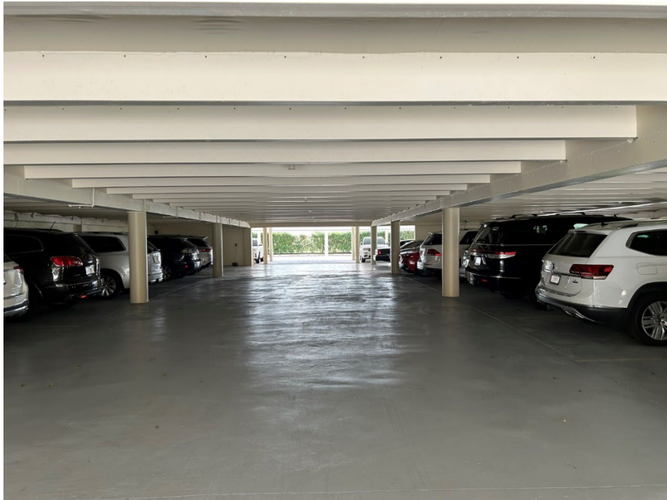
12. View of the parking garage.
