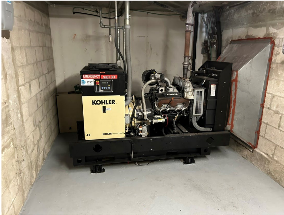
21. View of the generator located at the roof top.
