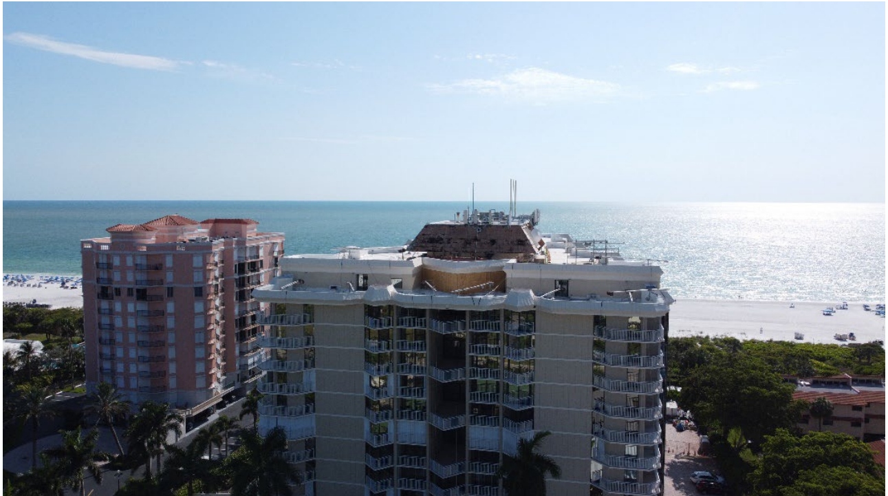
2. View of the roof line of the building.
