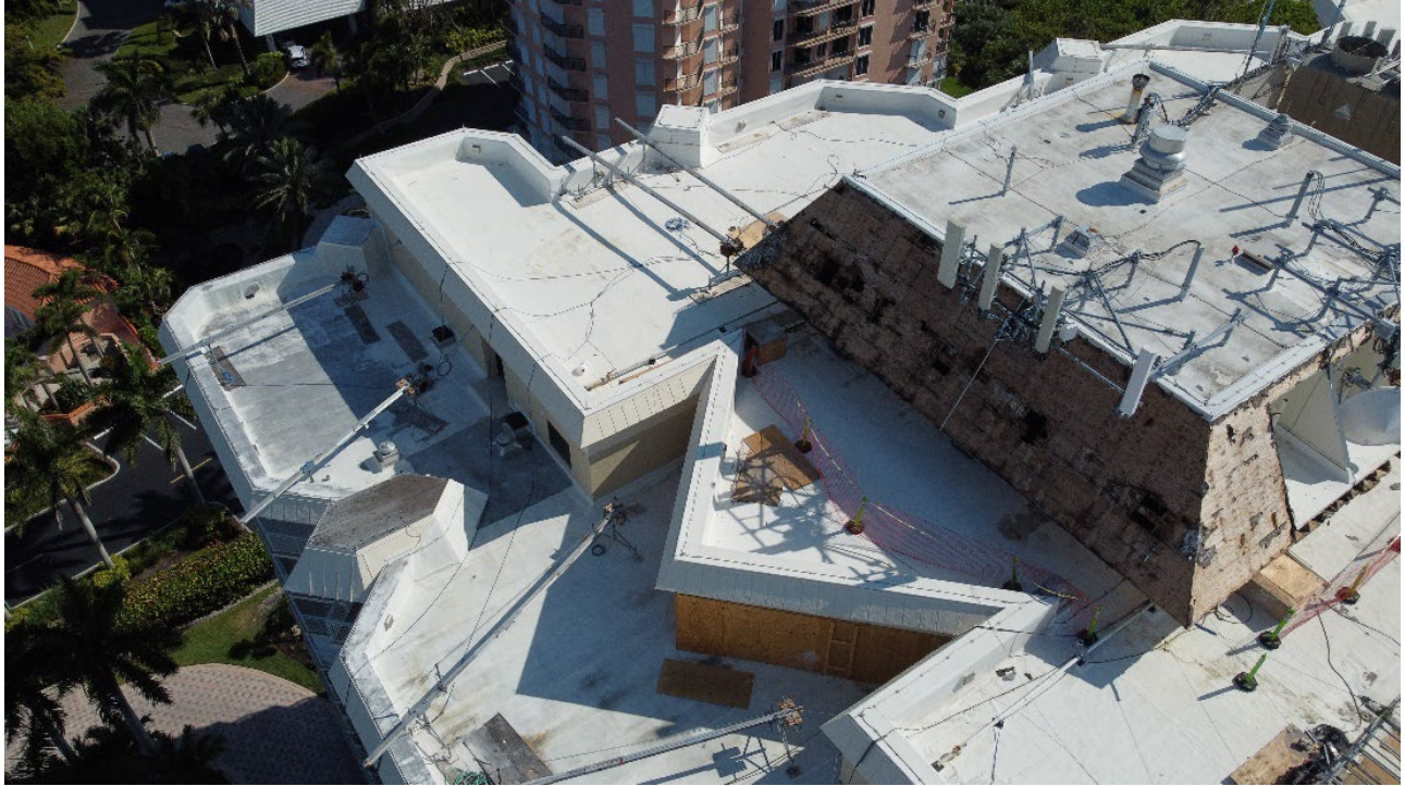
3. View of the work that is being performed on the terrace (middle roof section).
