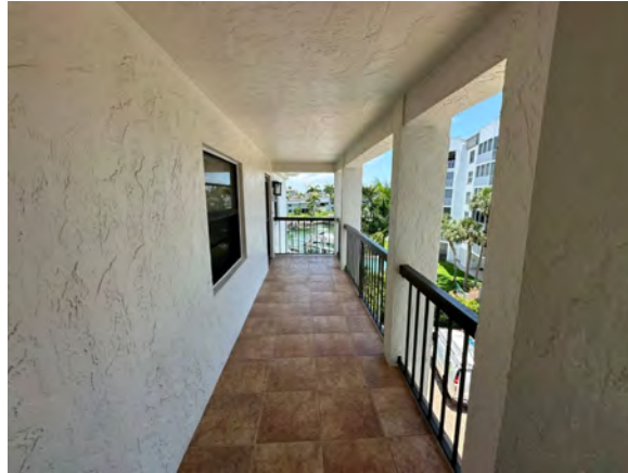
VIEW OF TYPICAL ELEVATED WALKWAY
