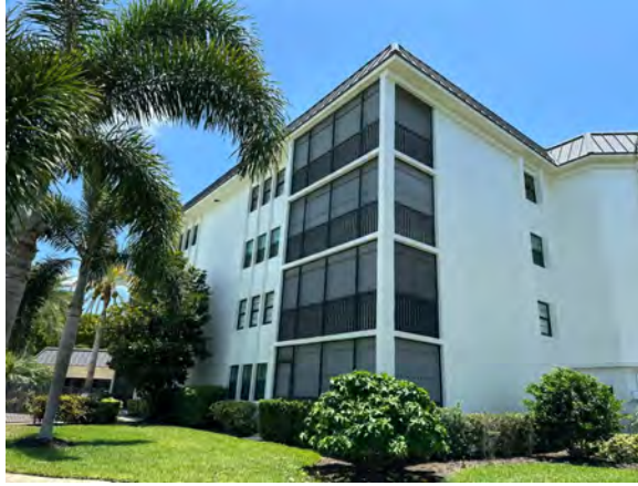
VIEW OF TYPICAL BALCONY
