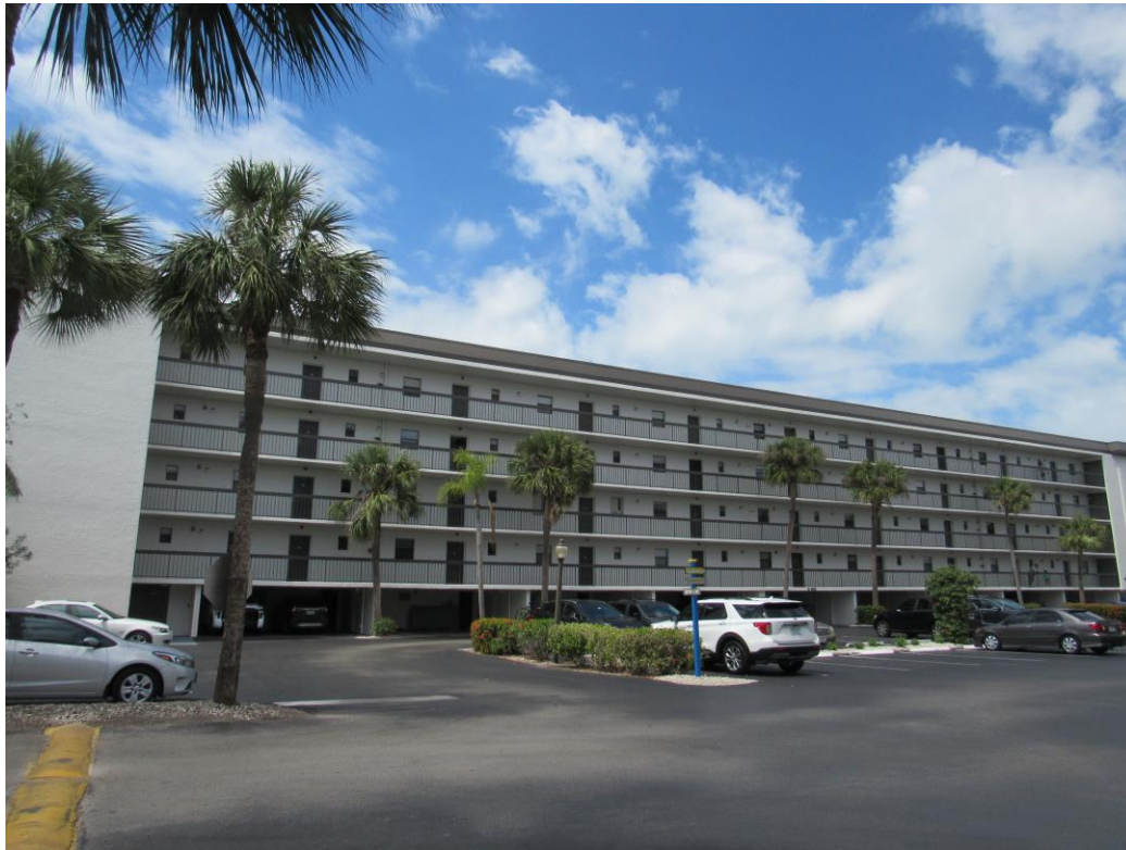
Overview of typical 5-story residential building at subject site.
