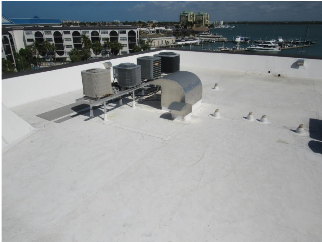
Overview of typical TPO roofing system at subject site.
