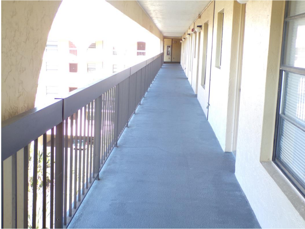
View of typical coated elevated walkway at subject site.
