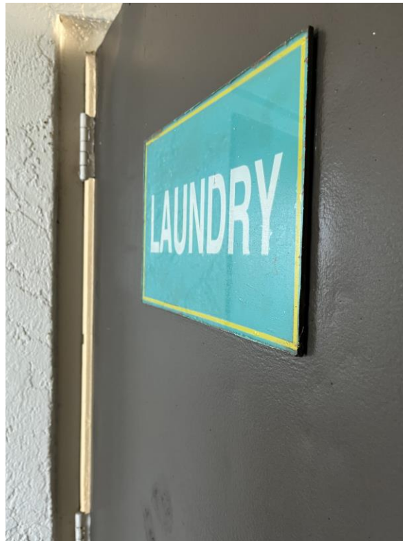
View of typical common area service door at subject site.
