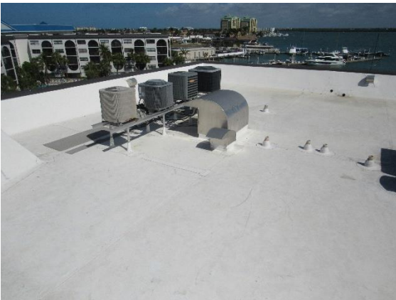
View of TPO roof system.
