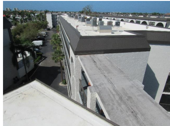
View of flat roof system.
