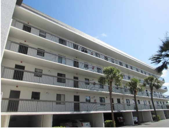
View of front of building.
