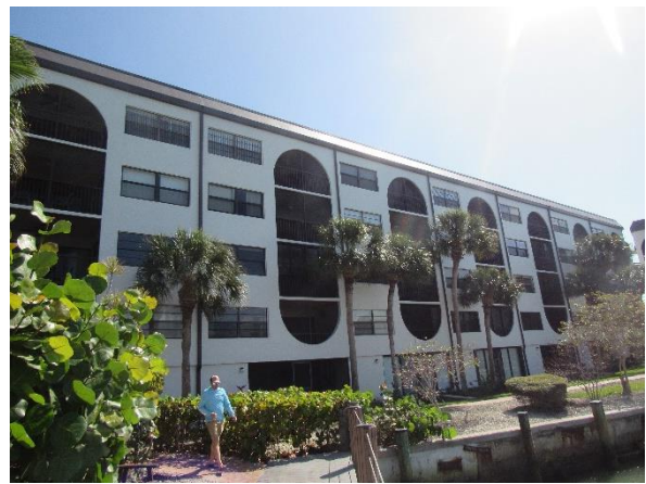
View of rear of building.
